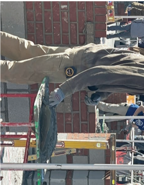
Ashton Sollars spreads mortar on his rowlock course.
