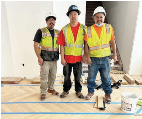
Hoem and Associates work at Stanford Mall.
