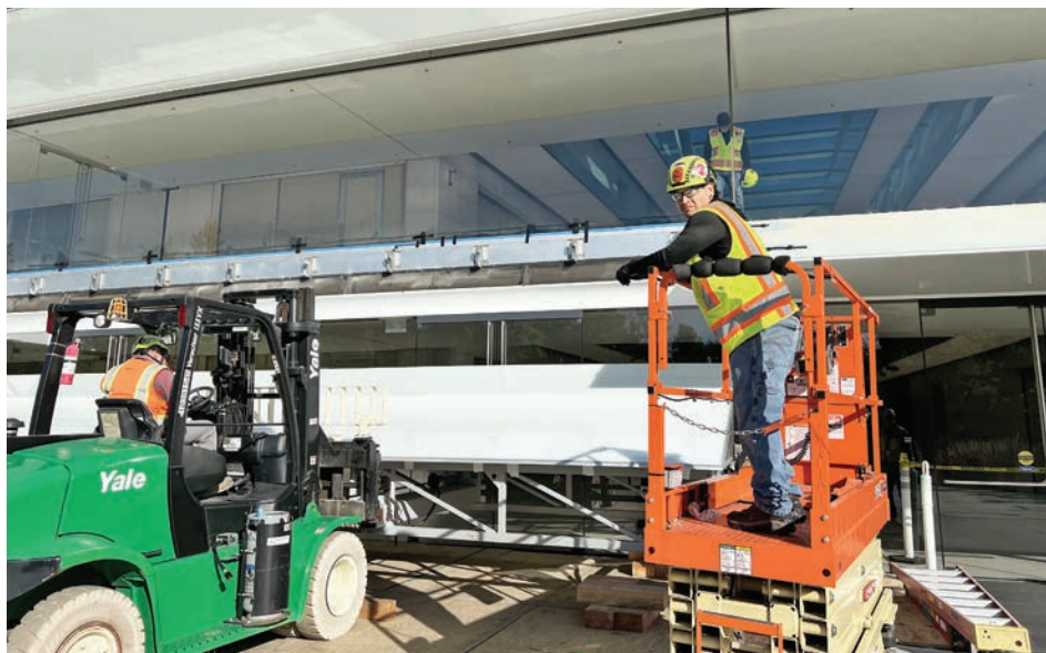
Steve Vargas, Jose Rocha, Jaime Rocha work on an Apple Campus canopy glass replacement.
