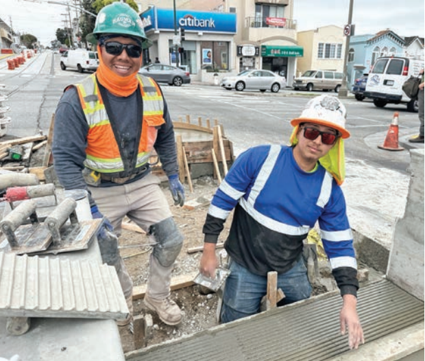
Local 300 cement masons Augustin Pinto and Daniel Rodriguez work with Bauman Landscaping at 19th Avenue and Taraval Street in San Francisco.
