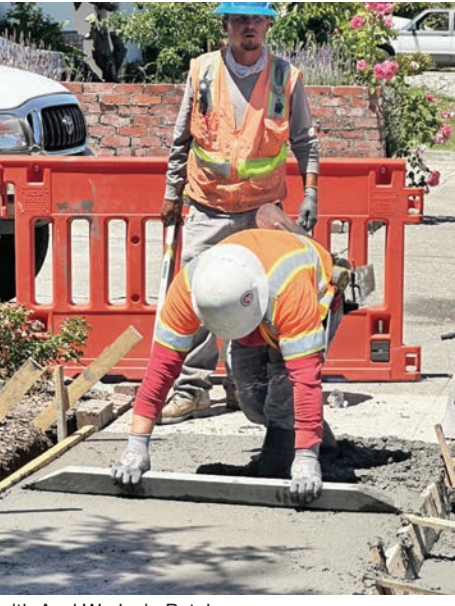
Local 300 cement masons work with Azul Works in Petaluma.
