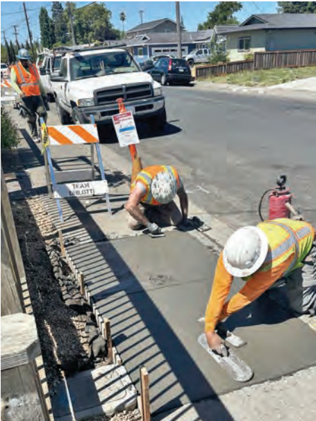
Local 300 cement masons work with Greg Nelson Concrete in Rohnert Park.
