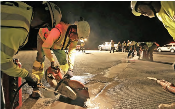
Local 300 cement mason Alex Rodriguez works with Granite Construction at the Charles Schulz Airport in Santa Rosa.
