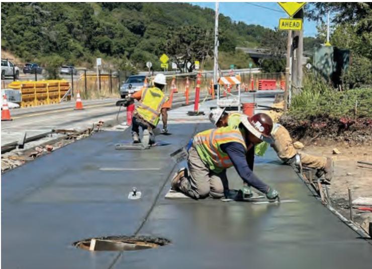
Local 300 cement masons work with Ghilotti Brothers Inc. in San Rafael.
