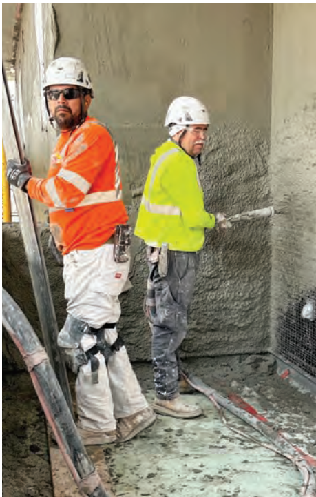
Local 300 plasterers with Anning Johnson Co. work on Yerba Buena Island.
