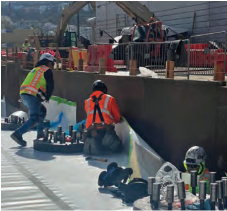
Local 40 members work on a below-grade waterproofing project at the SFPUC Biodigester jobsite in the Bayview.
