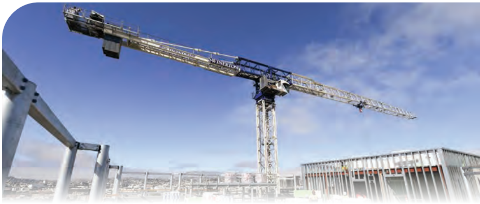
The 555 Bryant Street jobsite
