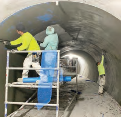
Local 300 plasterers work in a North Bay wine cave for Frey Plastering.
