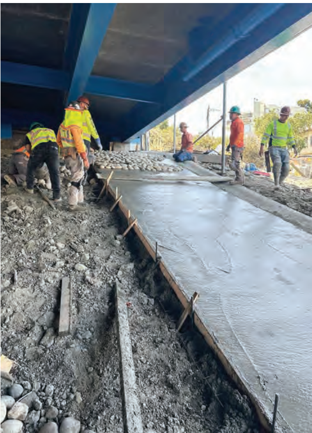
Local 300 cement masons work with Bauman Landscape and Construction beneath Highway 101 in San Francisco.
