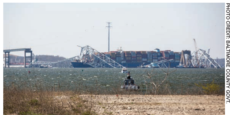
Baltimore's collapsed Key Bridge is seen on Friday, March 29, three days after a massive container ship hit the span, destroying it.
