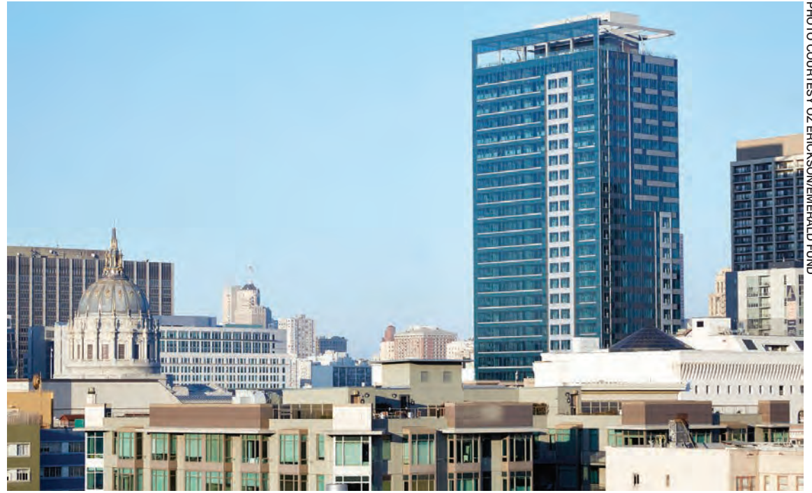
An example of a successful commercial-to-residential conversion in San Francisco, the tower at 100 Van Ness Avenue opened as an office building in 1974 and was converted to residential use in 2015, as seen here.
