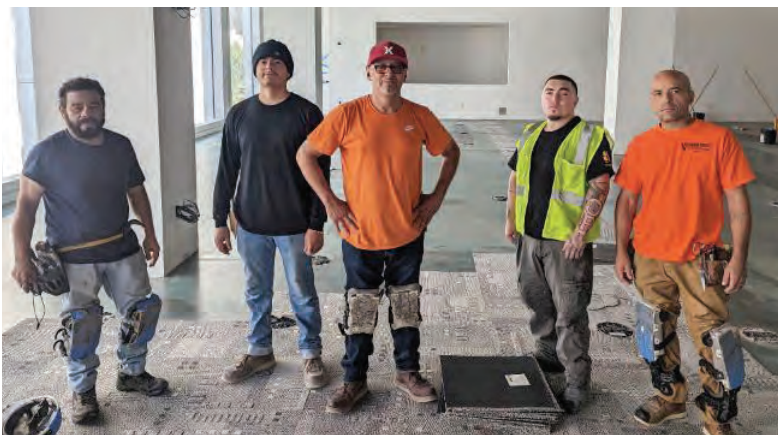
Golden State Floors workers are seen out on the job.
