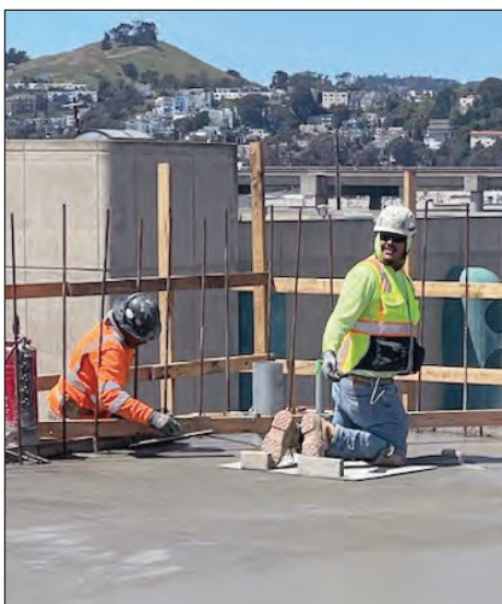
Local 300 cement mason Osmar Gambino Rivera works with R&S Construction at the Potrero Power Plant project on San Francisco's Central Waterfront.
