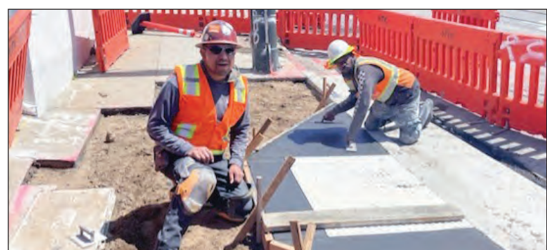
Local 300 cement masons work with On The Level Concrete at 19th Avenue and Taraval Street in San Francisco.
