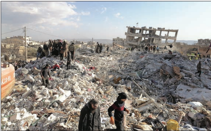
The sheer devastation from recent severe earthquakes in Western Asia and the Middle East is seen in Aleppo, Syria, on February 8.
