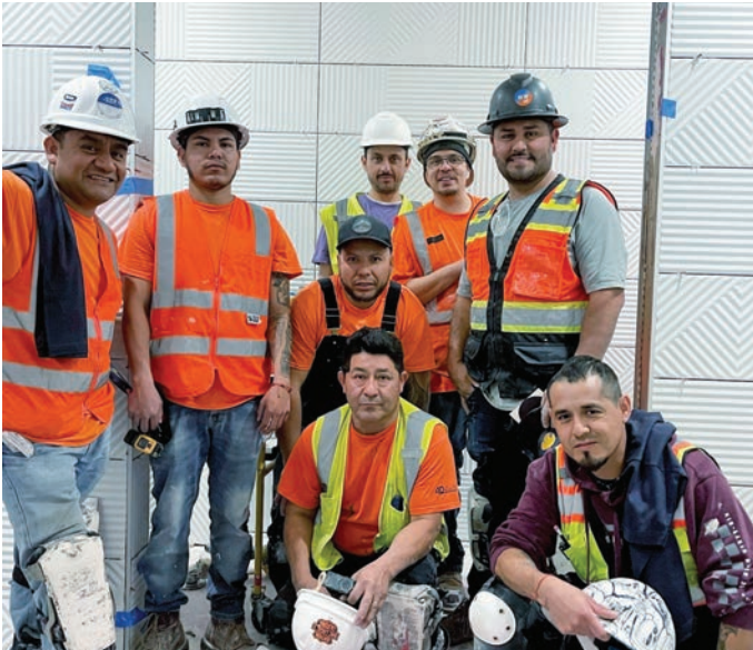
The Rinaldi Tile and Marble crew working at Google Plymouth in Mountain View
