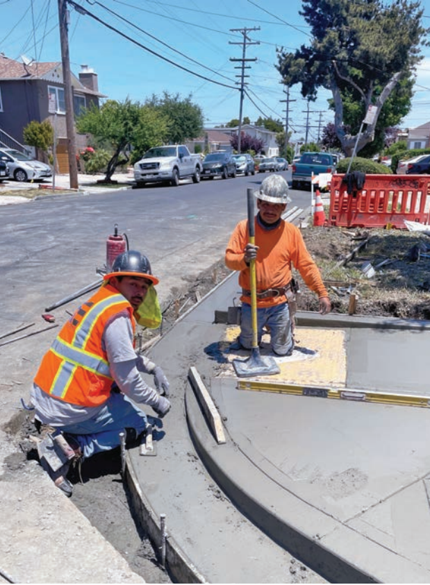
Local 300 cement masons who work with RK Engineering install new ADA-compliant ramps in San Bruno.
