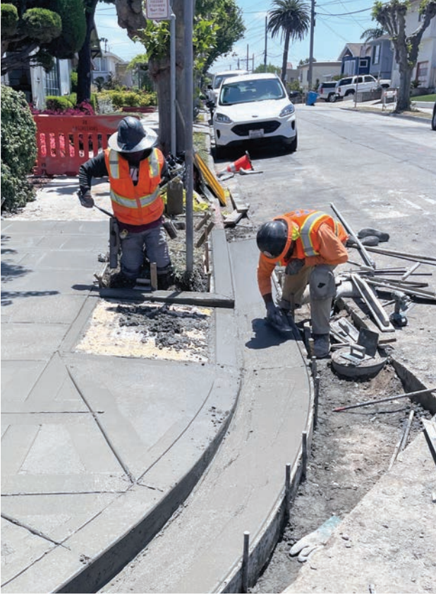
Local 300 cement masons who work with RK Engineering install new ADA-compliant ramps in San Bruno.
