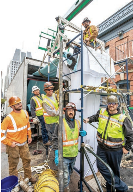
SF Public Utilities Commission workers from Local 261 are proud to serve you, San Francisco.
