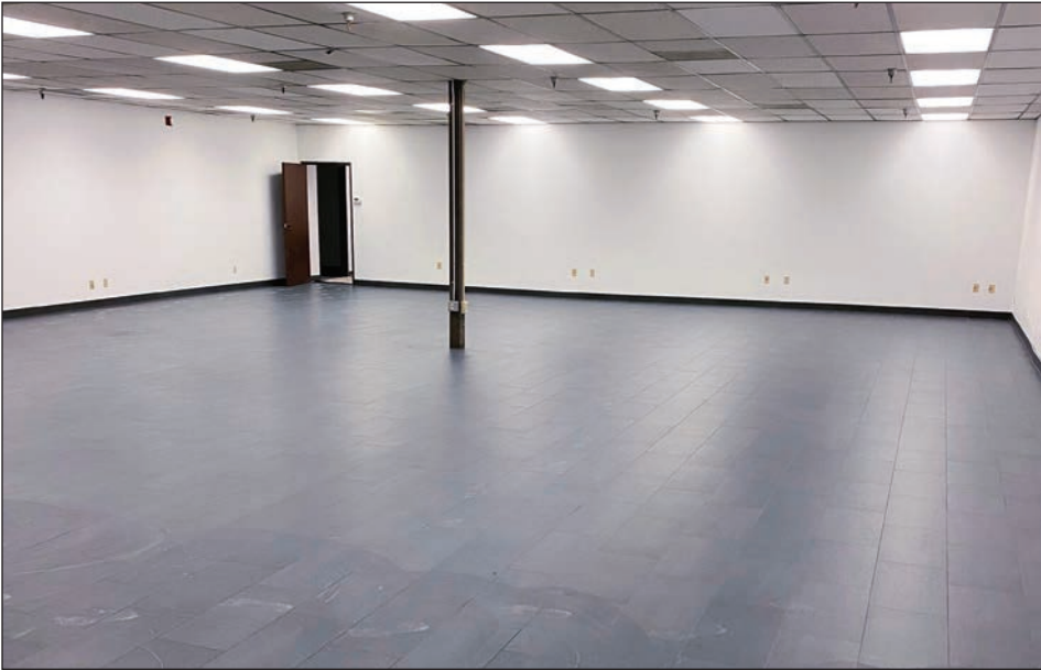
Thank you to all the BAC members who helped install tile at our new Sacramento Union Hall.
