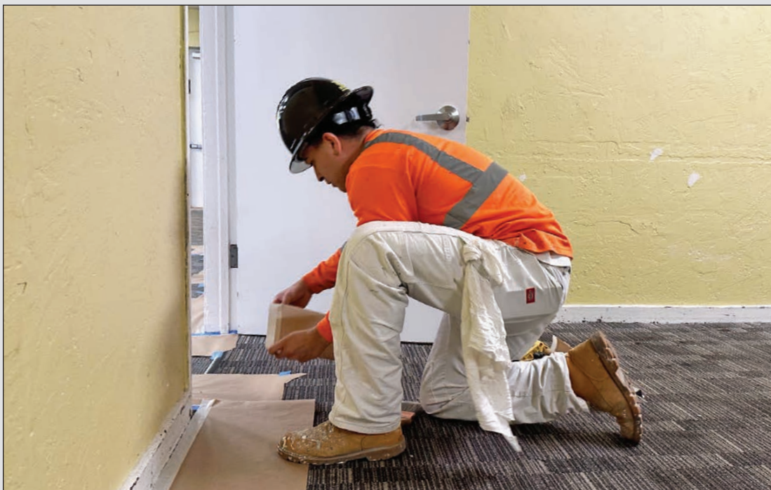
Jose Villanueva (Painters and Drywall Finishers Local 487) masks carpet in preparation for repairing and repainting.
