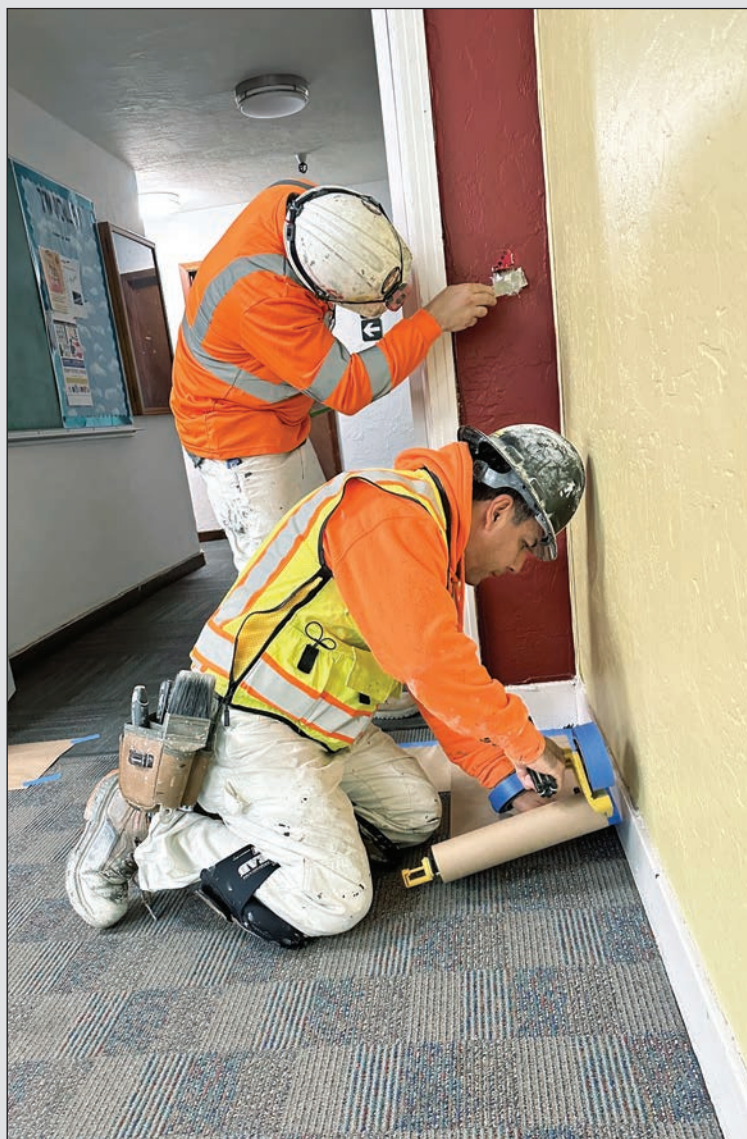
Jason Casas (Local 741), standing, and Jorge Ortega (Painters and Drywall Finishers Local 3), kneeling, spackle a hole and mask carpet.
