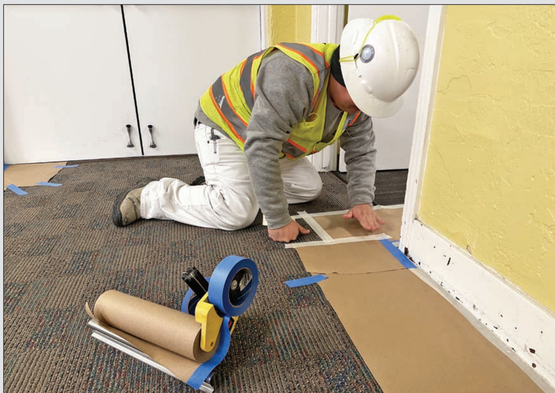
Salvador Hernandez (Local 741) masks carpet in preparation for repairing and repainting.
