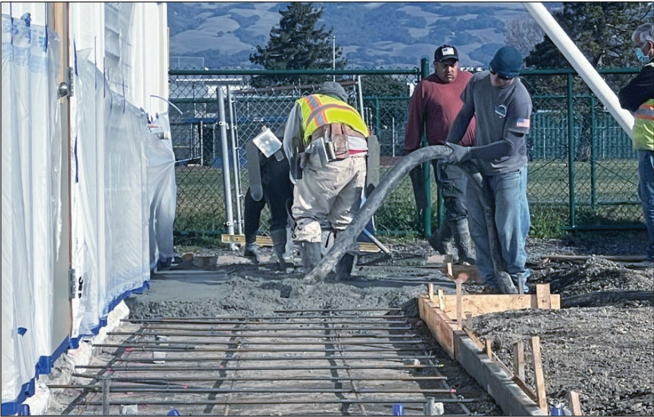
Local 300 cement masons at work in Petaluma.
