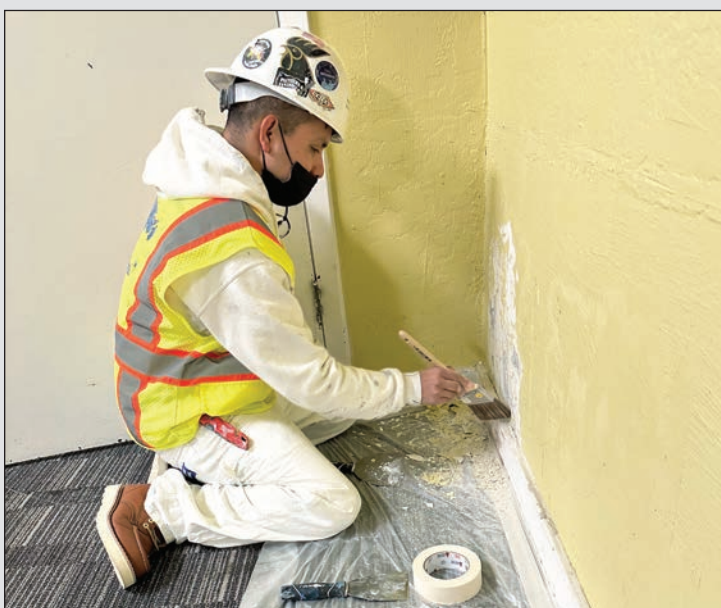
Jose Hernandez (Painters and Drywall Finishers Local 741) finishes sanding a patch.
