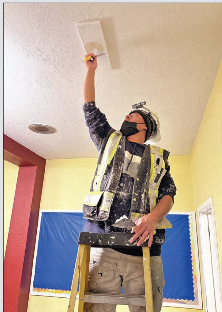
Artemio Gramajo (Painters and Drywall Finishers Local 913) spackles holes in preparation for painting the ceiling.
