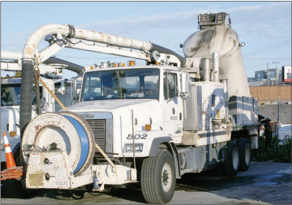
The plumbers of U.A. Local 38 are instrumental in keeping the City's sewers up and running during powerful storms. Vacuum trucks such as the one pictured here are crucial tools for the job.
