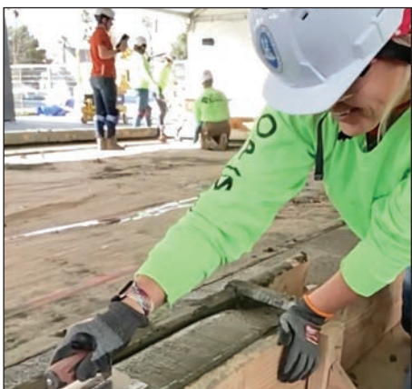
Kilah Engelke works in the OPCMIA Steel Edge Women's demonstration at this year's World of Concrete event in Las Vegas.
