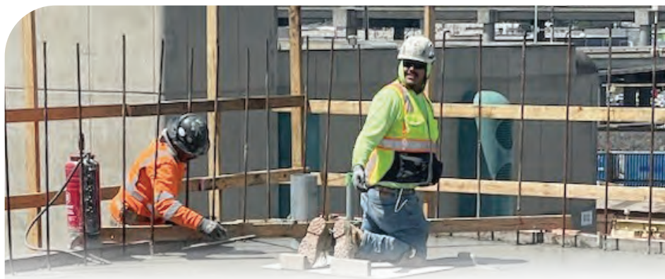
Local 300 member Osmar Gambino Rivera at the Potrero Power Plant jobsite in May
