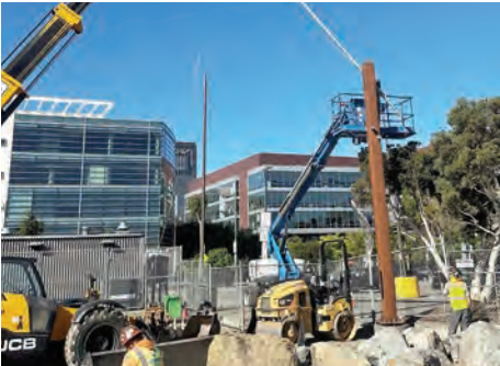
Local 6 member Jessie Nungaray (bottom right) hoists a light post on a recent project.
