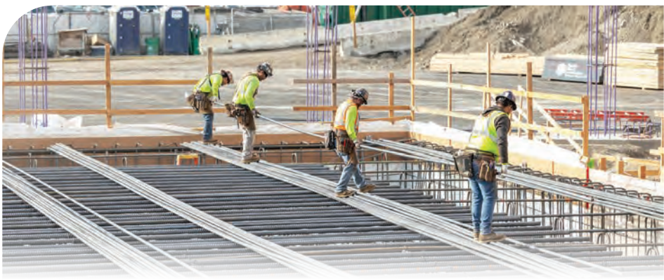
Local 261 members fit rebar at the Mission Rock jobsite in 2022
