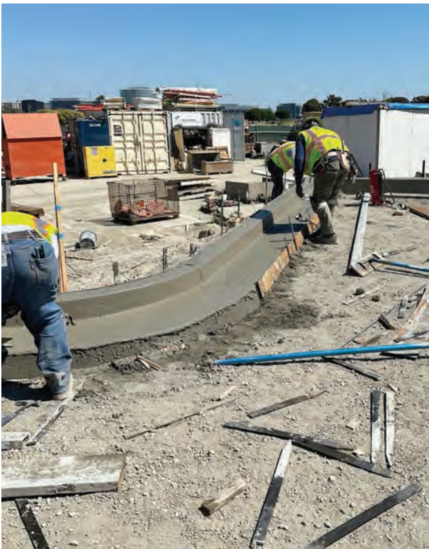
Local 300 cement masons work with Shaw and Sons in Brisbane.
