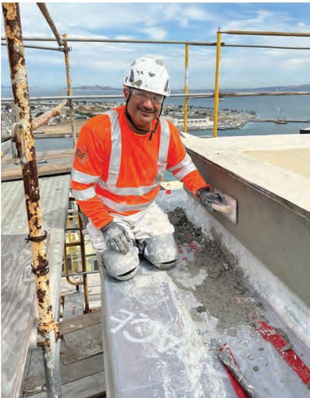
Local 300 plasterer Rogelio Carrillo works with Anning and Johnson at the Yerba Buena Island Residences.
