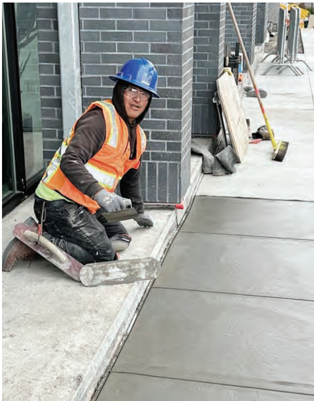
Local 300 cement mason apprentice Ivan Ayra works with Minerva Construction in San Francisco.
