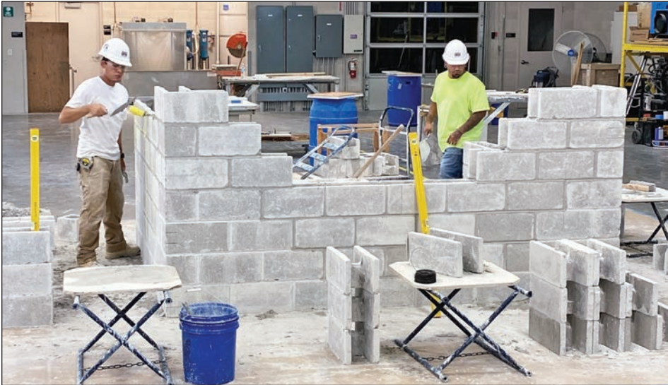
Pre-apprentices Erik Mendoza and Hubert Tercero learn the basic of laying brick and block.
