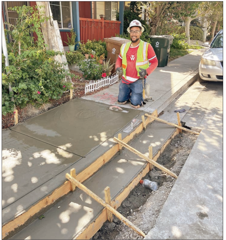
Luis Sánchez is a Local 300 cement mason 95% apprentice.
