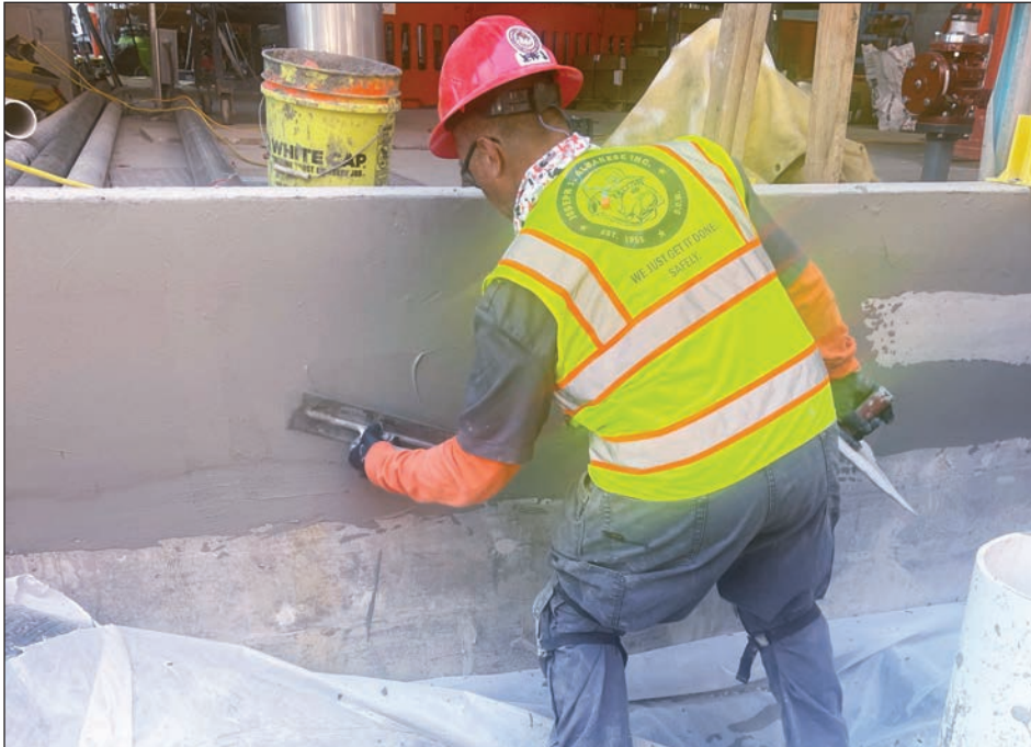
Local 300 cement mason journeyman Jeff Jessap works at Mission Rock Parcel A.
