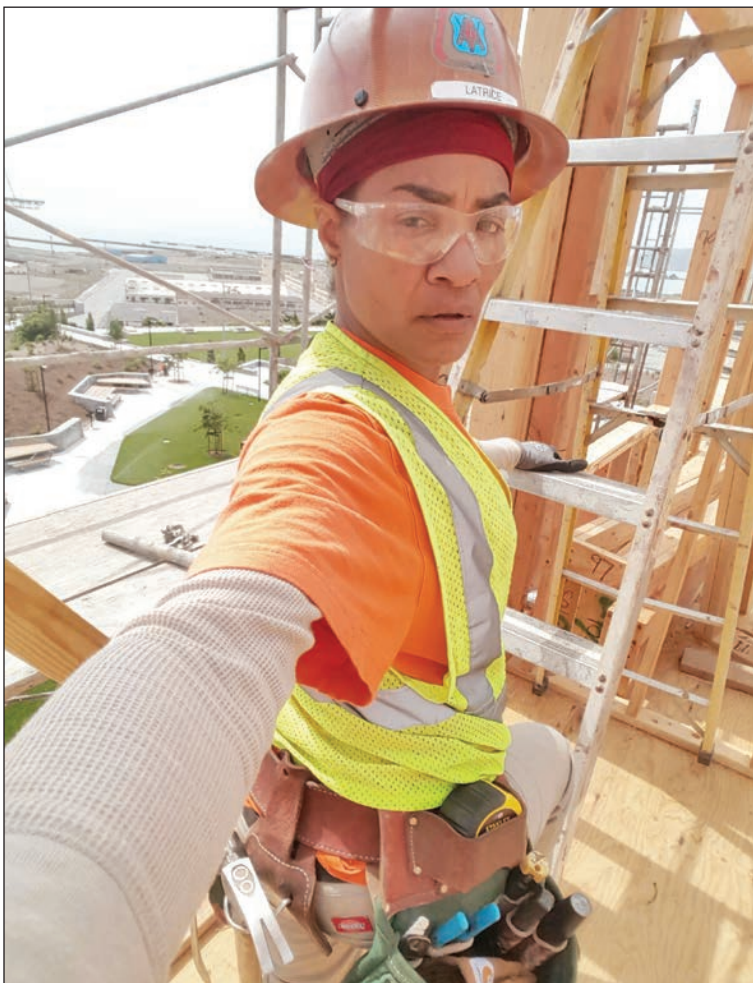
Latrice Madaris at the Hunters Point Shipyard jobsite.
