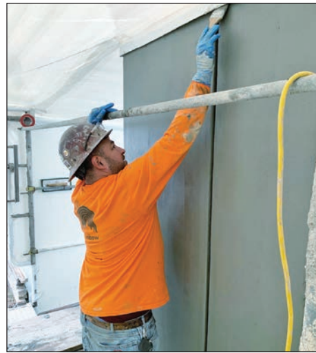
A Local 40 member works on a restoration job at UCSF for contractor Rainbow Waterproofing and Restoration.
