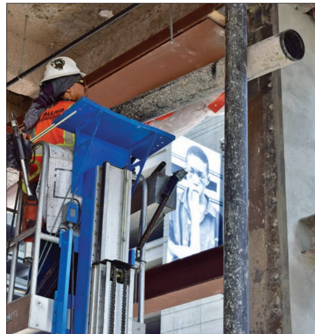
A Local 483 member installs a fire sprinkler system pipe at the Mexican Museum jobsite in April 2020.
