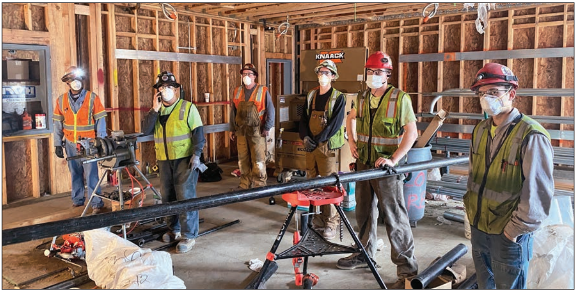
Local 483 members prepare to install pipes for a fire sprinkler system at the Michelle Obama School in Richmond shortly after construction workers were declared essential during the pandemic in 2020.
