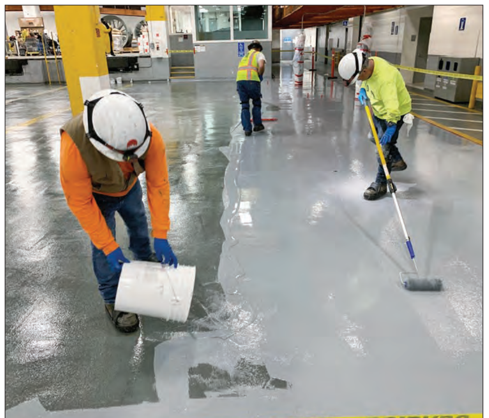
Urethane coating is applied to a floor by the Rainbow Waterproofing and Restoration crew.
