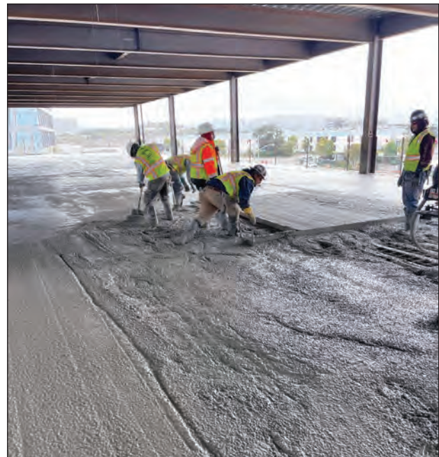
Cement masons with Dolan Concrete work on the Kilroy project in Oyster Point.
