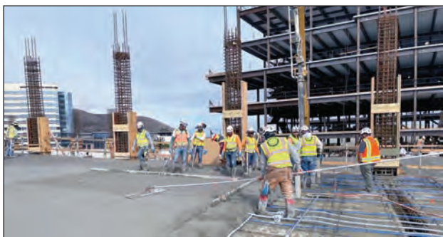
Cement masons with J.J. Albanese work on GOP Phase 5 in Oyster Point.
