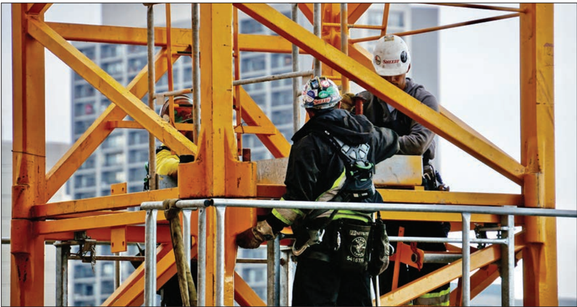
San Francisco operating engineers work to erect a tower crane on a jobsite in spring 2020.
