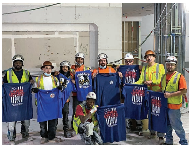
BAC members with American Terrazzo working at Park West in Downtown San Francisco.
