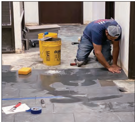
Field Rep Jordan Mondragon lays tile at the new Sacramento office.
