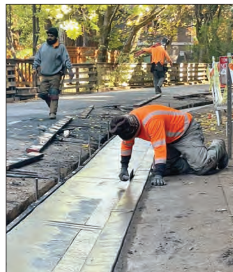
Antonio Espinosa, a Local 300 cement mason, works in Mill Valley.
