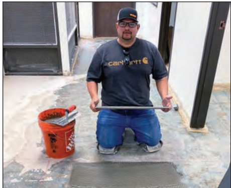
Local 3 Vice-Chair and organizer Dave Tafoya lays tile at the new Sacramento office.
