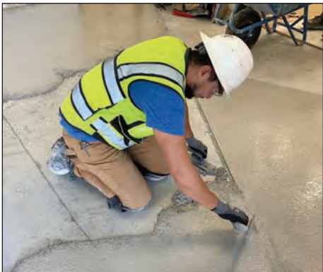
Apprentice Noel Anzora-Arias places terrazzo in the lobby of the new Sacramento office.
