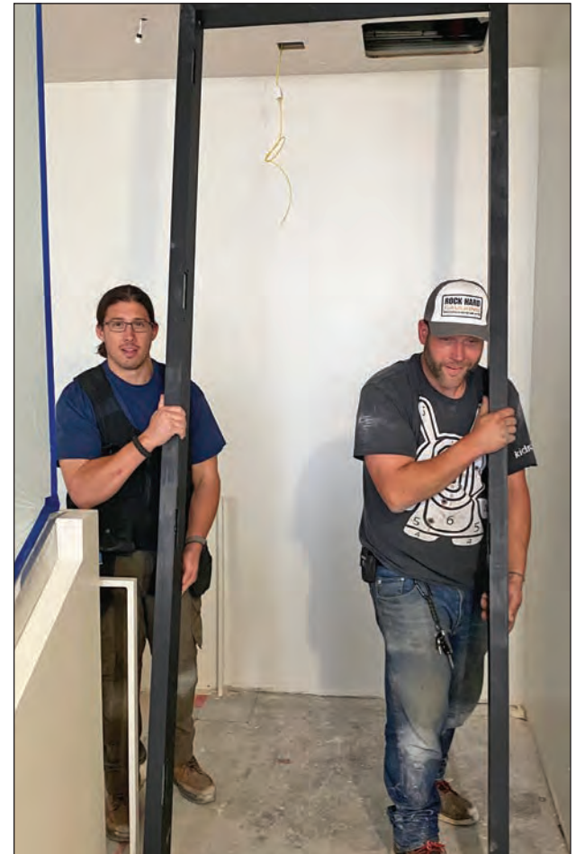
Michael Brannan and Ken Clark transport a window frame on the jobsite at One Maritime.
