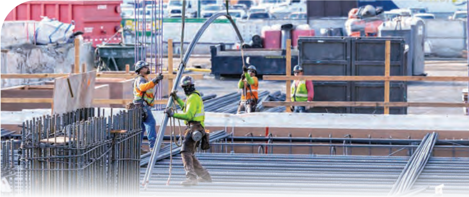
Fitting rebar at Mission Rock
