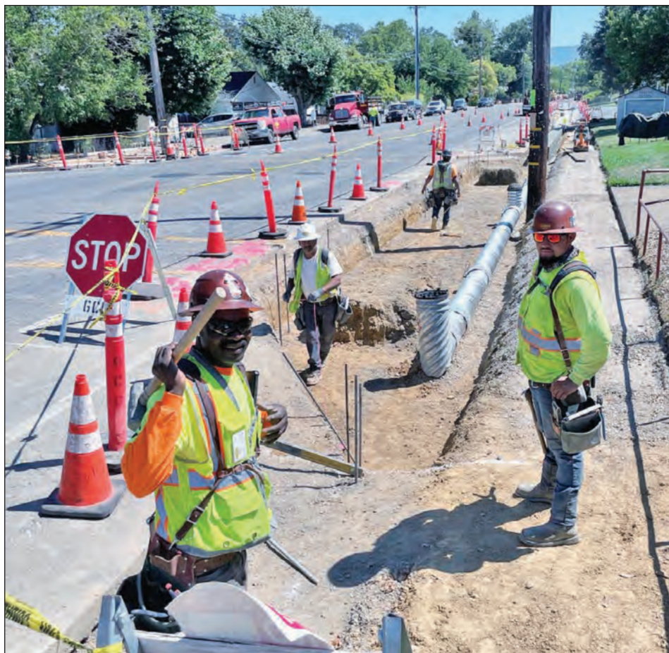
Local 300 cement masons Gilles Doumate and Cuauhtemoc Calderon work on a jobsite for Ghilotti Construction in Ukiah.
