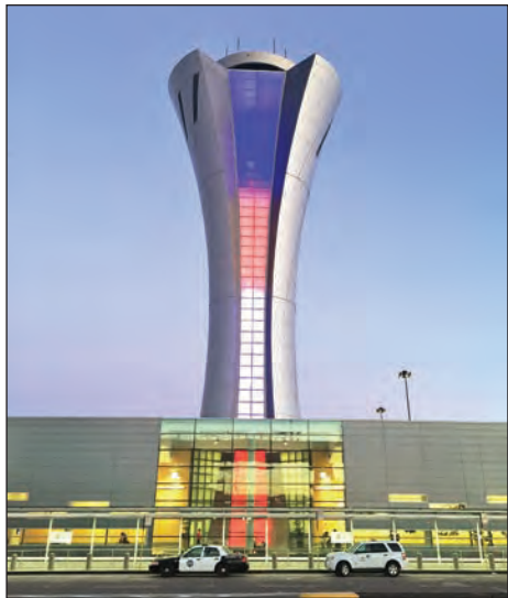
A new air traffic control tower was built under the SFO PLA and opened in 2016.
