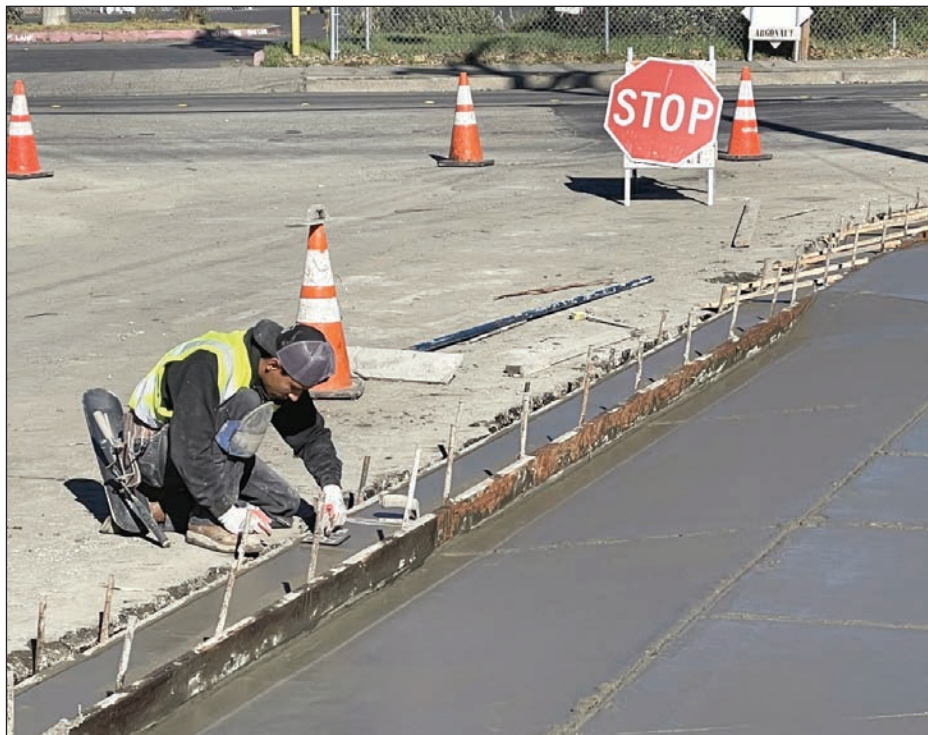
Local 300 cement mason apprentice Marco Montenez working in Santa Rosa.
