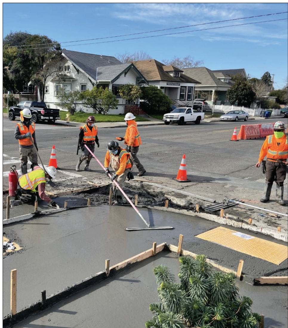
Local 300 cement masons on the job with Azul Works in Petaluma.
