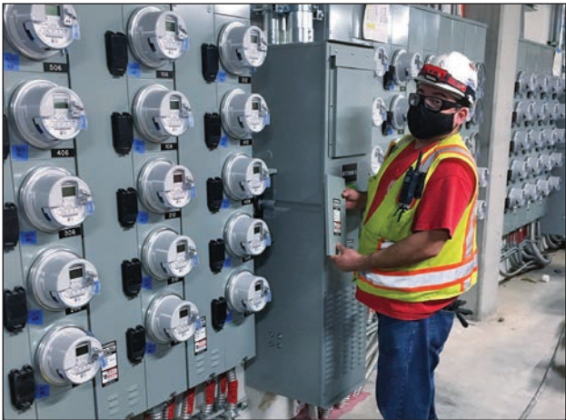
IBEW Local 6 inside wireman foreman Carlos Salazar works on the electrical service indoors in a Yerba Buena Island residential project on Sept. 1, 2021.
