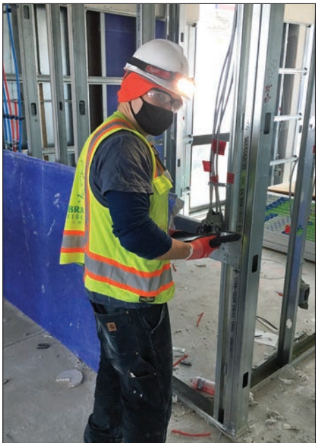
IBEW Local 6 inside wireman apprentice Jared Nelson rings out a residential unit at a residential project on Yerba Buena Island on Sept. 1, 2021.
