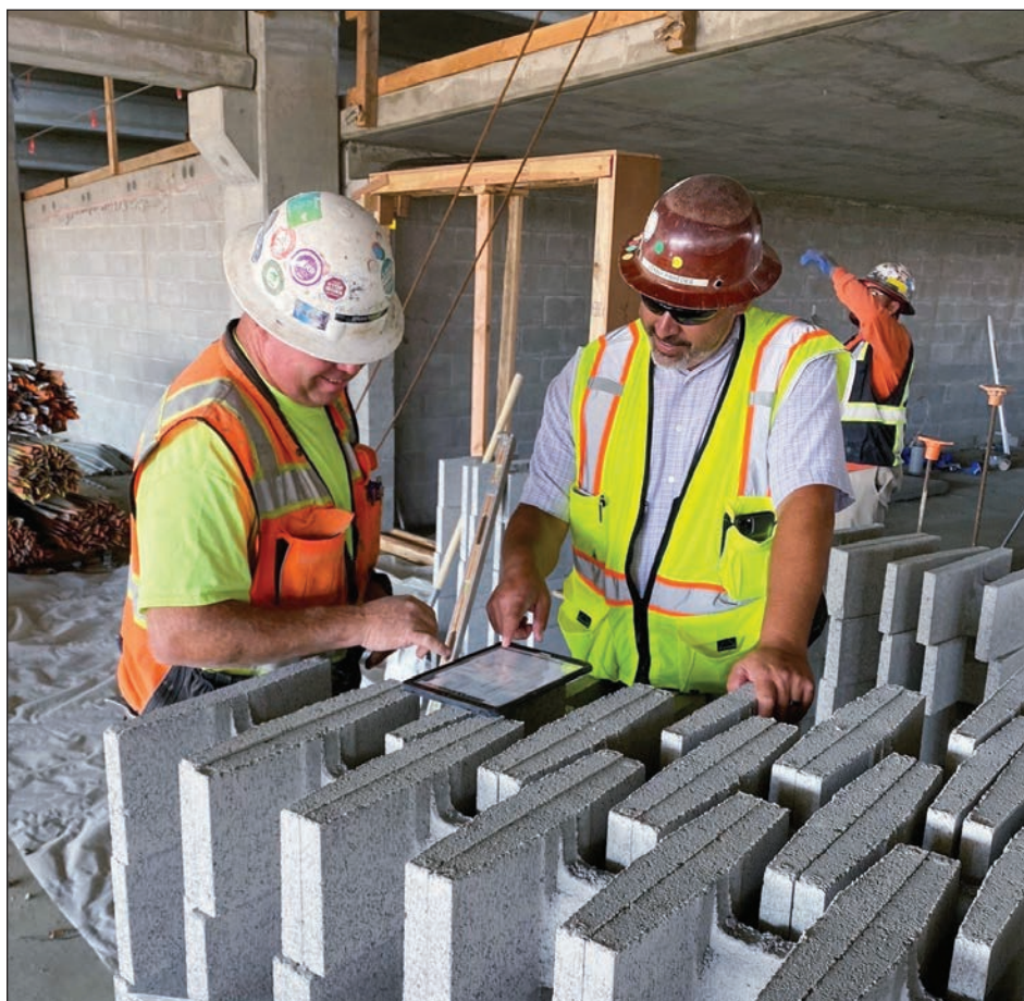
(L-R) Brian Reeve and Lenny Paredes looking at plans at the Richards Blvd. office complex parking structure.
