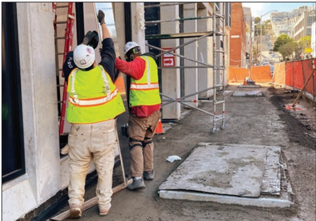
Glaziers Local 718 apprentice Tony Roberto (foreground, left) and journeyman Kimani Goodwin (background, right) install architectural panels on the outside of the 88 Broadway building in San Francisco in 2021.
