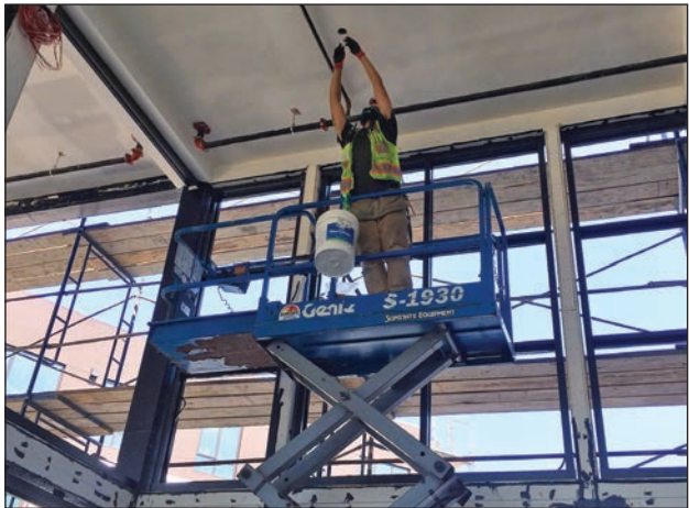
IBEW Local 6 inside wireman foreman Joey Chow works on lobby lighting for a Yerba Buena Island residential project on Sept. 1, 2021.
