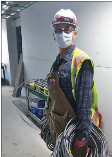
IBEW Local 6 journeyman inside wireman McJullian Jaochico works indoors wiring units on a project on Yerba Buena Island on Sept. 1, 2021.
