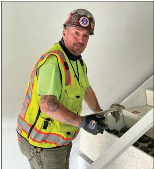
Gerry Mansfield installs pre-cast terrazzo steps.
