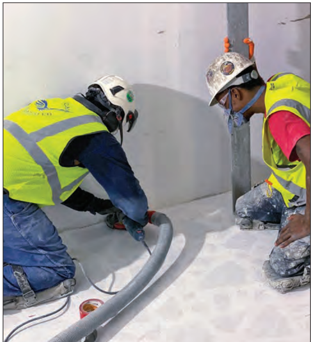
Thomas McCoy and Malik Salam edge-grinding the terrazzo at the walls.
