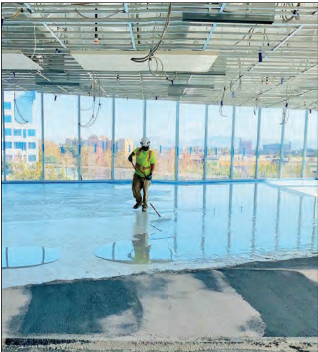
Wily Tizoc spreads crack isolation membrane.
