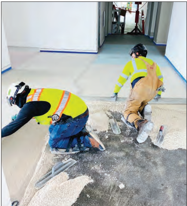
Alfonso Alvarado and Brian Dohring install a sand-and-epoxy mortar bed.
