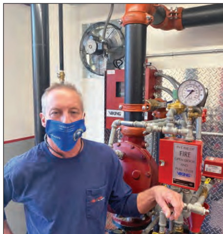
Ralph Farber, an eighth-period apprentice, U.S. Air Force veteran, and Sprinkler Fitters Local 483 member, is currently completing the union's apprenticeship program.
