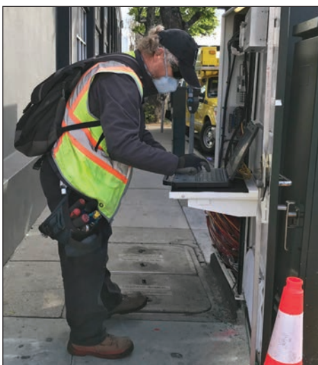
Alan Coughlan, traffic signal electrician for SFMTA and member of IBEW 6, uses a laptop to program accessible pedestrian signal buttons with custom verbal messages for people with hearing impairments.
