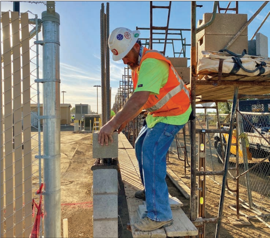
Matt Kirkes, laying block for JD Wait Masonry at the Newman Water Treatment Plant.
