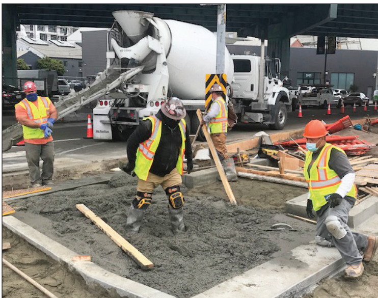
San Francisco Public Works cement shop crew members construct ADA-compliant curb ramps in the city during the pandemic.
