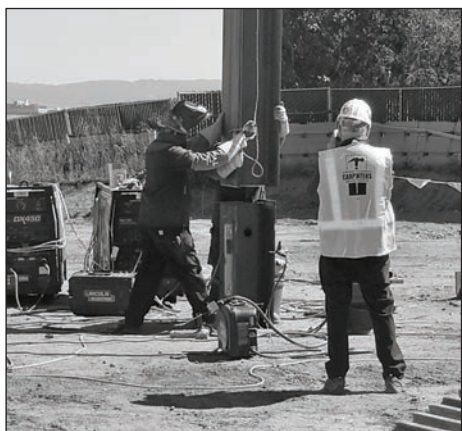
A Carpenters Magazine reporter photographs Local 34 members splicing H-Pile.
