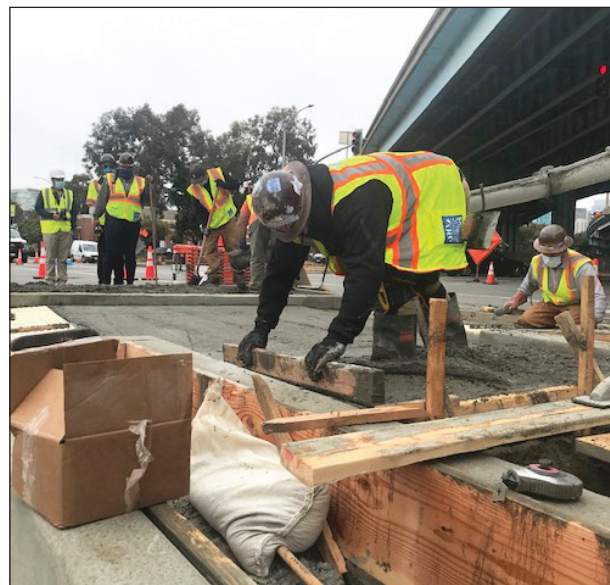
San Francisco Public Works cement shop crew members construct ADA-compliant curb ramps in the city during the pandemic.
