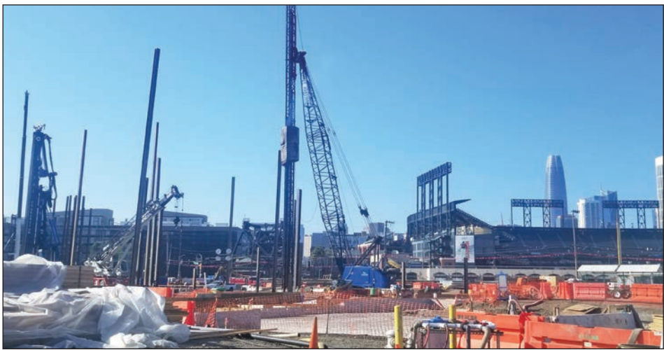
Two Foundation Constructors Inc. pile-driving crews splice and drive H-piles in Seawall Lot 337. The work advances the Mission Rock development project.
