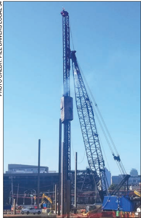
Members of Pile Drivers Local 34 and Operating Engineers Local 3 drive steel H-piles in the Mission Rock development project.
