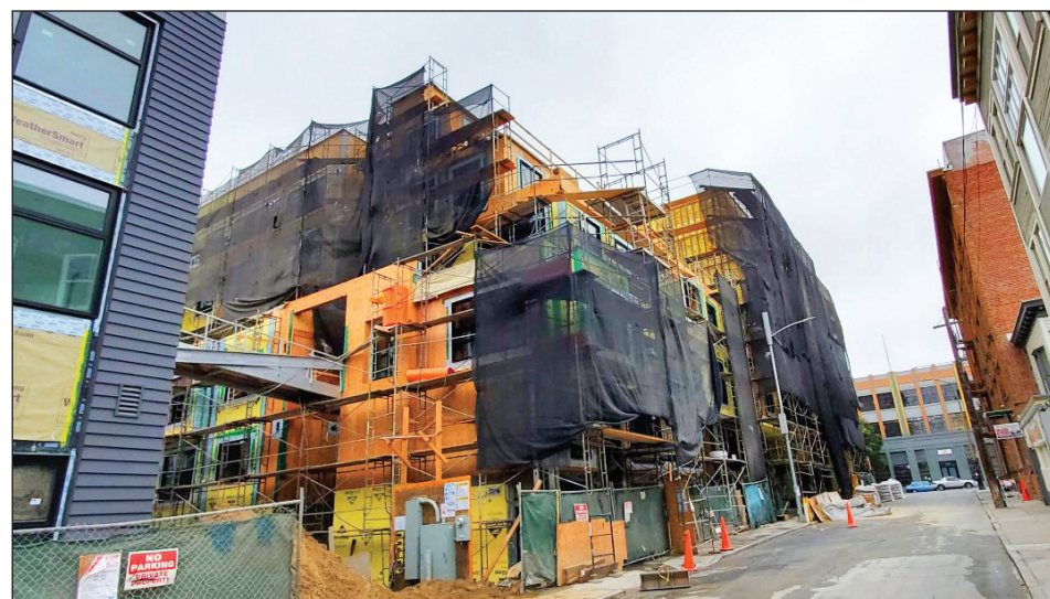
A top-to-bottom non-union residential construction project in San Francisco appears desolate on a late afternoon in mid-July.
