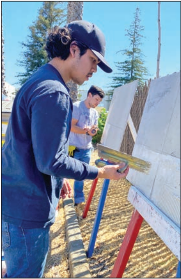
Two San Joaquin cohort students practice prepping the cement board for tile-laying.
