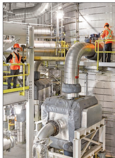
Boilermakers work on a carbon capture project in Alberta, Canada.
