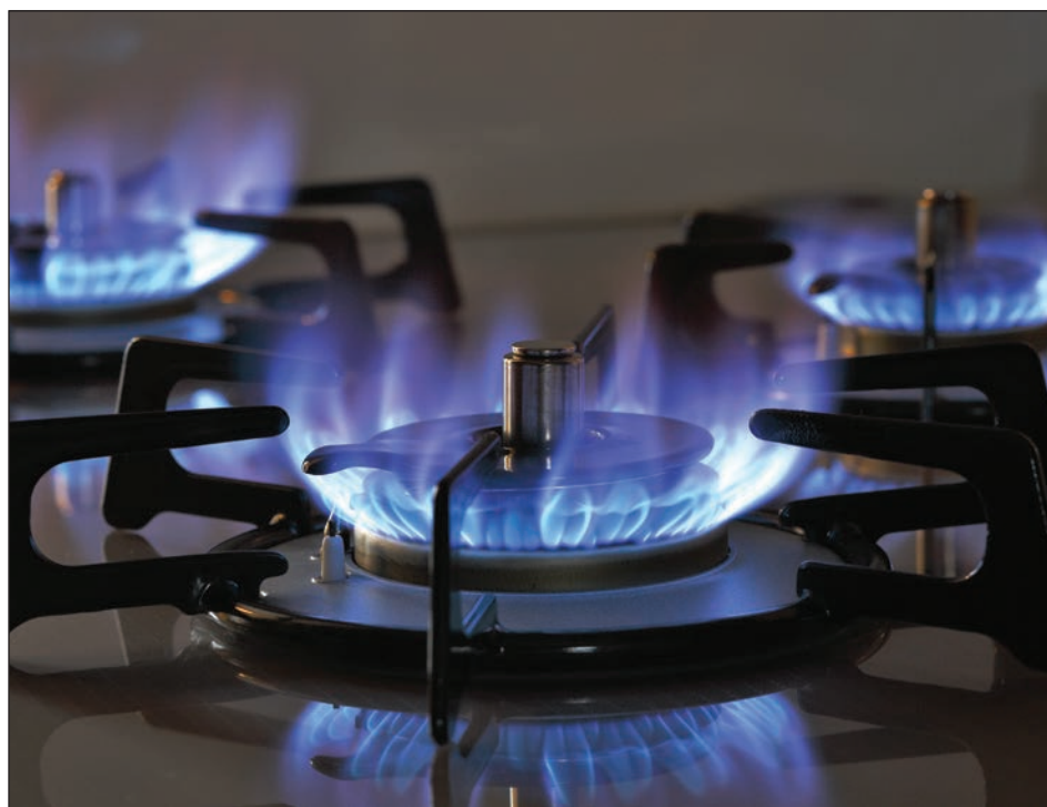
San Francisco will ban the use of natural gas in stoves, heaters and other appliances in new buildings beginning June 1, 2021.
