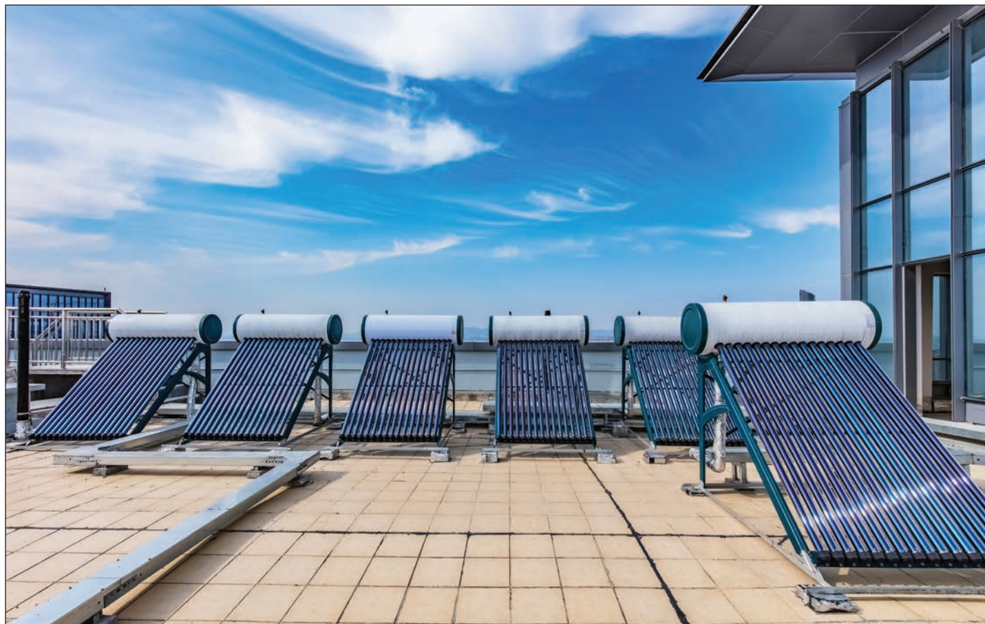
The installation of solar water heaters in high-rise residential and other buildings could help recover work for union plumbers.
