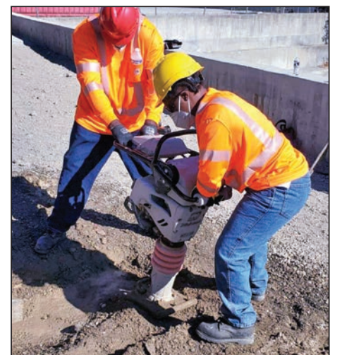
Darius Coleman (left) and Jimesse Powell (right) fill a hole and compact the ground with a jumping jack in a Laborer's Training Center class. This hands-on, trade-specific training with union members took place in fall 2020.
