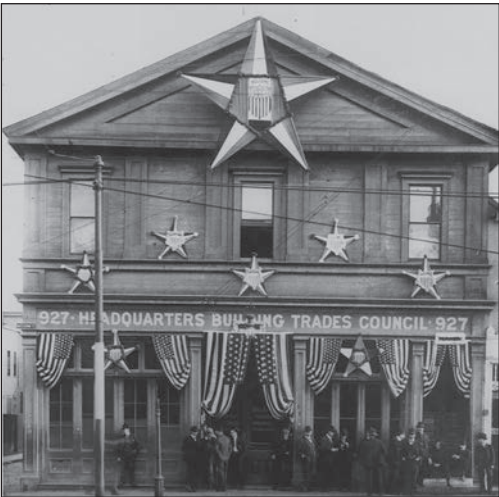
The San Francisco Building Trades Council’s headquarters, circa 1905.
