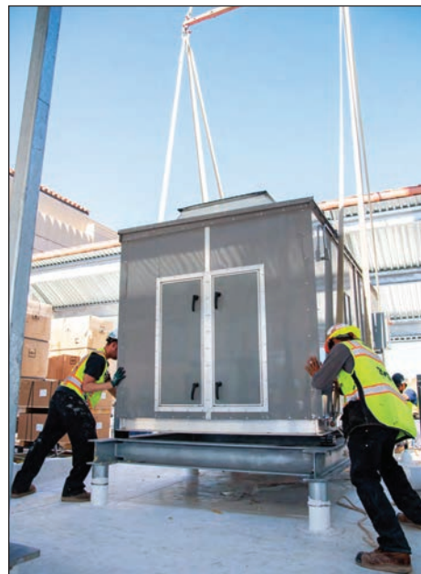
Sheet Metal Workers Local 104 members on the Escondido Village jobsite put together elements of a building providing new housing for Stanford University graduate students on Stanford's campus in October 2019.
