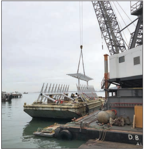
New sheet metal work at the San Francisco Ferry Terminal goes up in October 2018. The eventual installation of the canopy shown here was completed at one of multiple new ferry portals by members of Brown Sheet Metal from Local 104.
