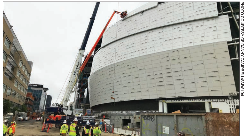
The "mega-panels" that enclose the exterior of the Golden State Warrior's Chase Center in San Francisco were fabricated by union sheet metal workers in the United States and installed by Sheet Metal Workers Local 104 members.
