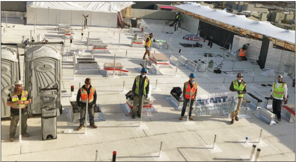
Sheet Metal Workers Local 104 members on a Bay City Mechanical job break from installing the HVAC and architectural sheet metal on a nine-story affordable housing project in the Mission to stand for a photo in 2019.
