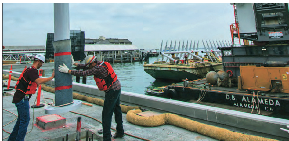
Members of Sheet Metal Workers Local 104 install a canopy at the San Francisco Ferry Terminal in October 2018.
