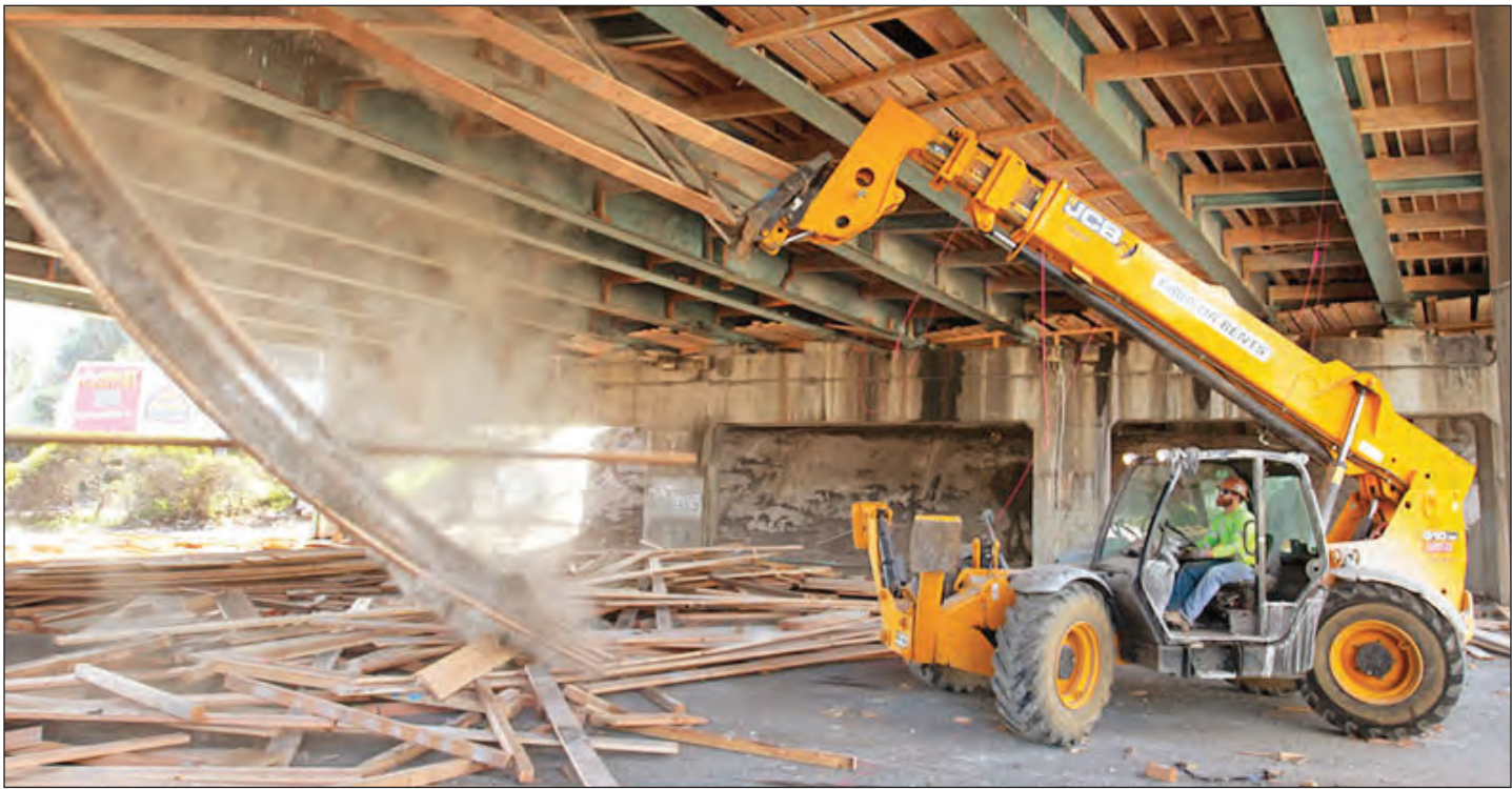
If the infrastructure bill becomes law, a significant increase will occur in federally funded infrastructure projects, such as CalTrans’s Alemany overpass replacement, seen here in May 2020.
