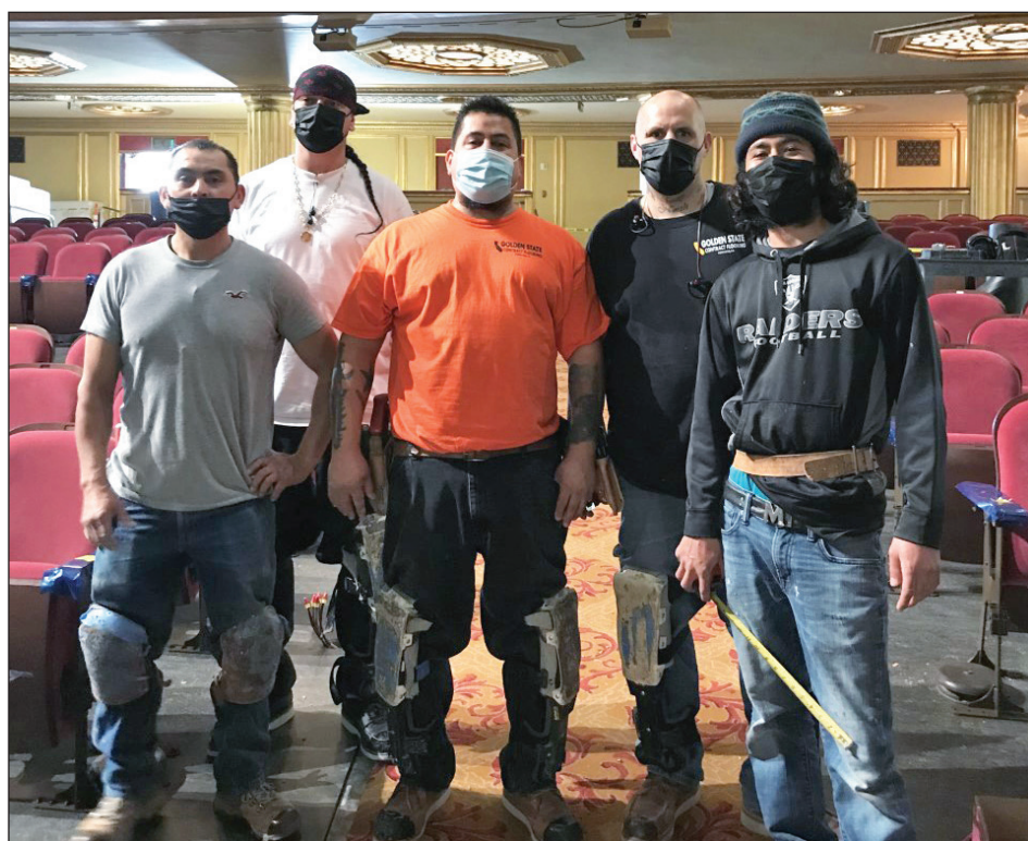
Golden State Flooring installing carpet at the San Francisco Opera House.
