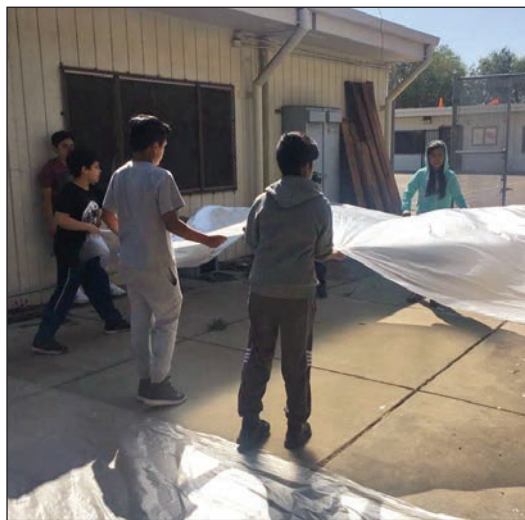
A group of kids work together to lay out plastic sheeting during park construction.
