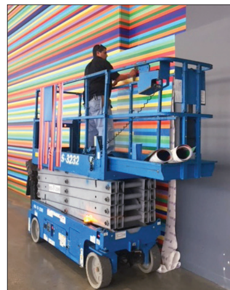
Journeyperson Frank Ramirez of Sign Display Local 510 installs graphic decoration on a wall at the Moscone Convention Center in July 2018.
