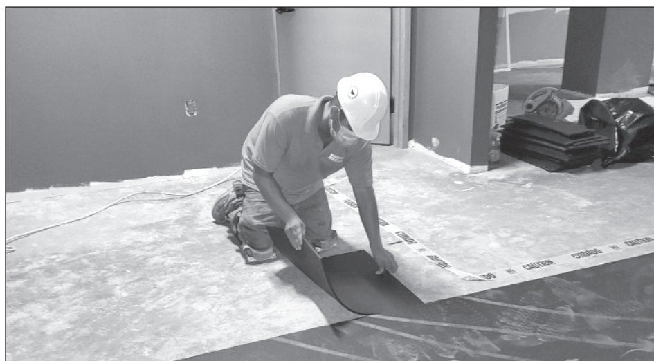
Michael Guerrero installing rubber tile.
