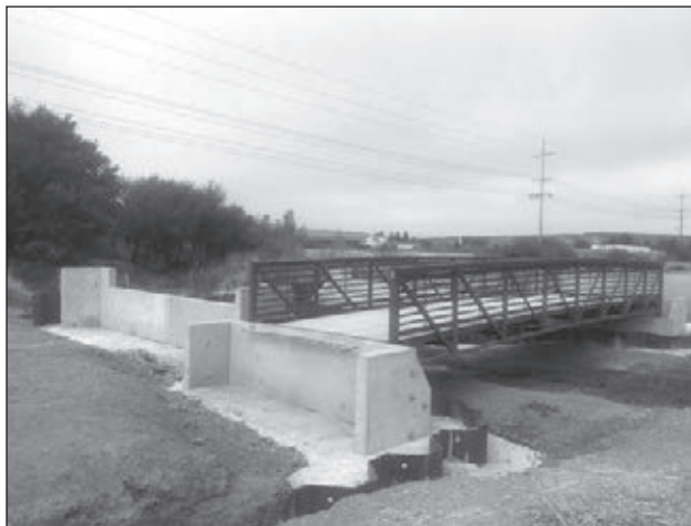
Pedestrian Bridge for SMART High Speed Rail worked on w Local 300 Cement Masons.
