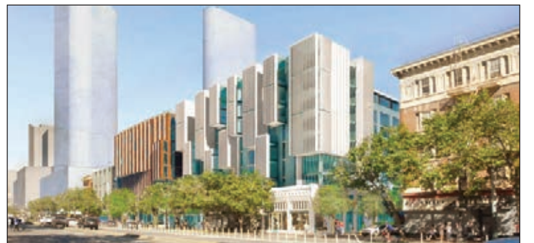
In July, Local 38 Plumbers & Pipefitters broke ground on a new headquarters and development at 1629 Market Street.
