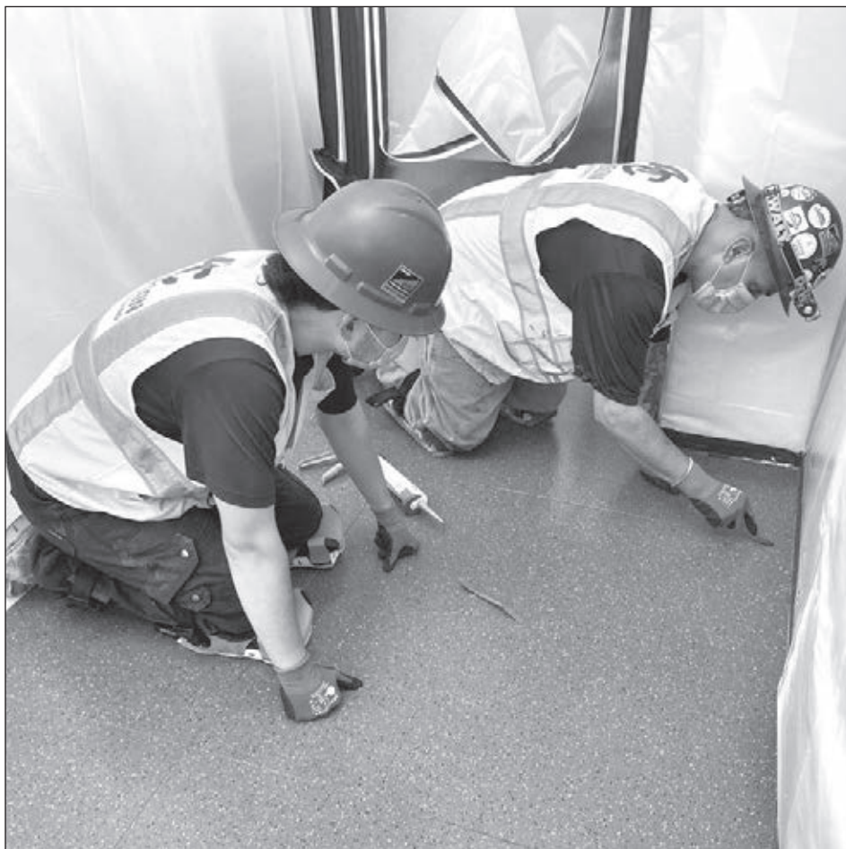
1st period Angel Santana and master installer Mario Herrera cold welding Nora tiles.
