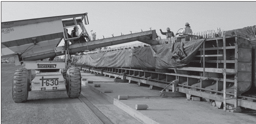
Brother Juan Sanchez oversees the pouring of a Bridge Girder while Brother Kevin Allen assists.
