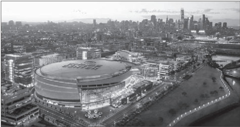
Once shovels hit the ground, the Golden State Warriors’ plan to construct a 13-story complex with a 129-room hotel, 20,000 square feet of retail and 21 condos will involve at least 600 union construction workers over a two-year construction period.
