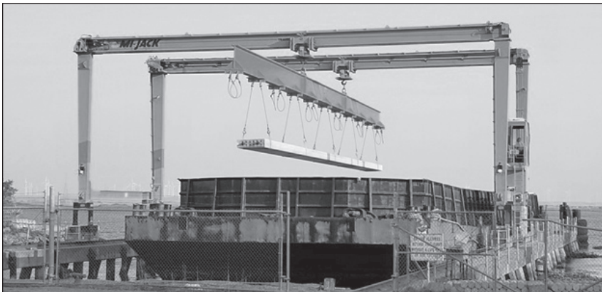
One of many concrete sheets being loaded on a barge, destined for Yerba Buena Island.
