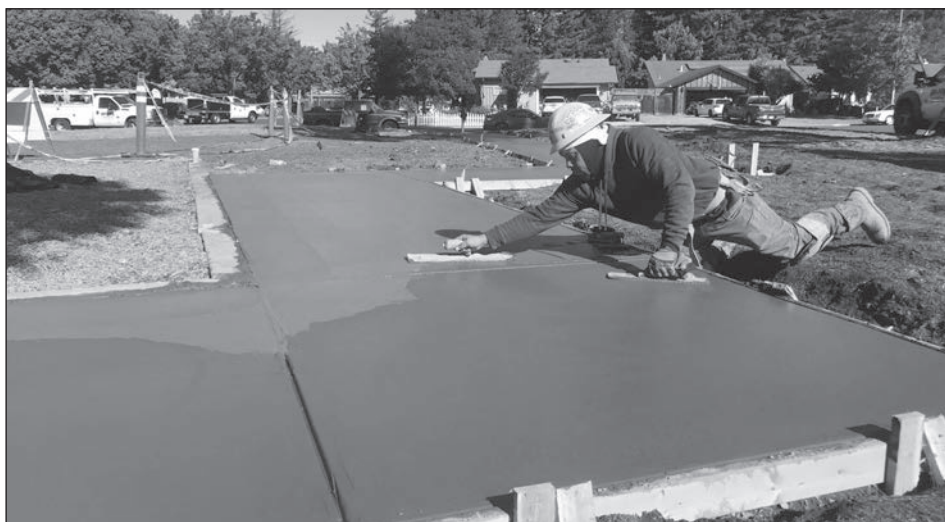
TOP: #300 Cement Mason Anthony Walker troweling sidewalk in Rohnert Park for Nelson Construction.
