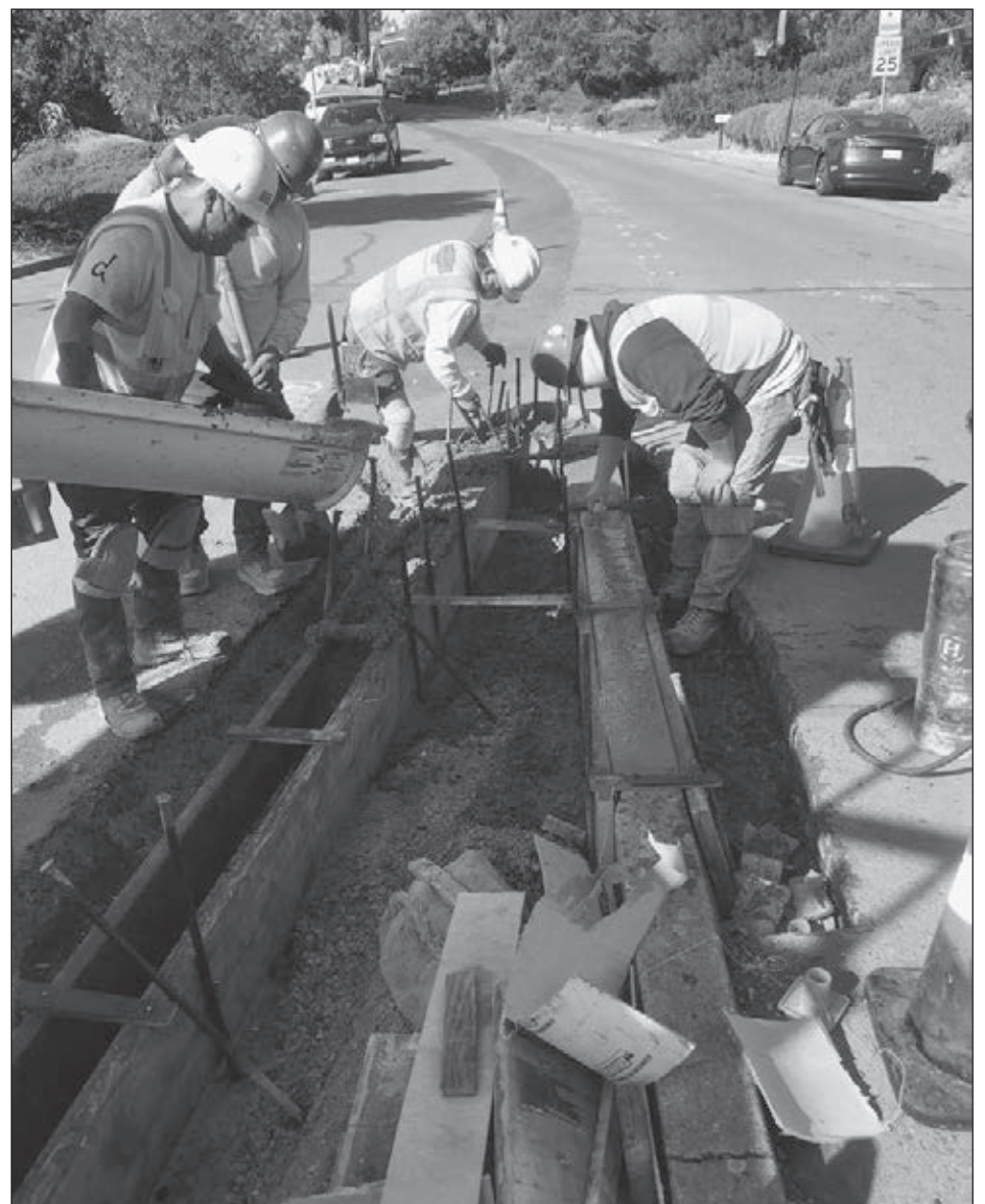
RIGHT: #300 Cement Masons with Ghilotti Construction pouring curb in Santa Rosa.
