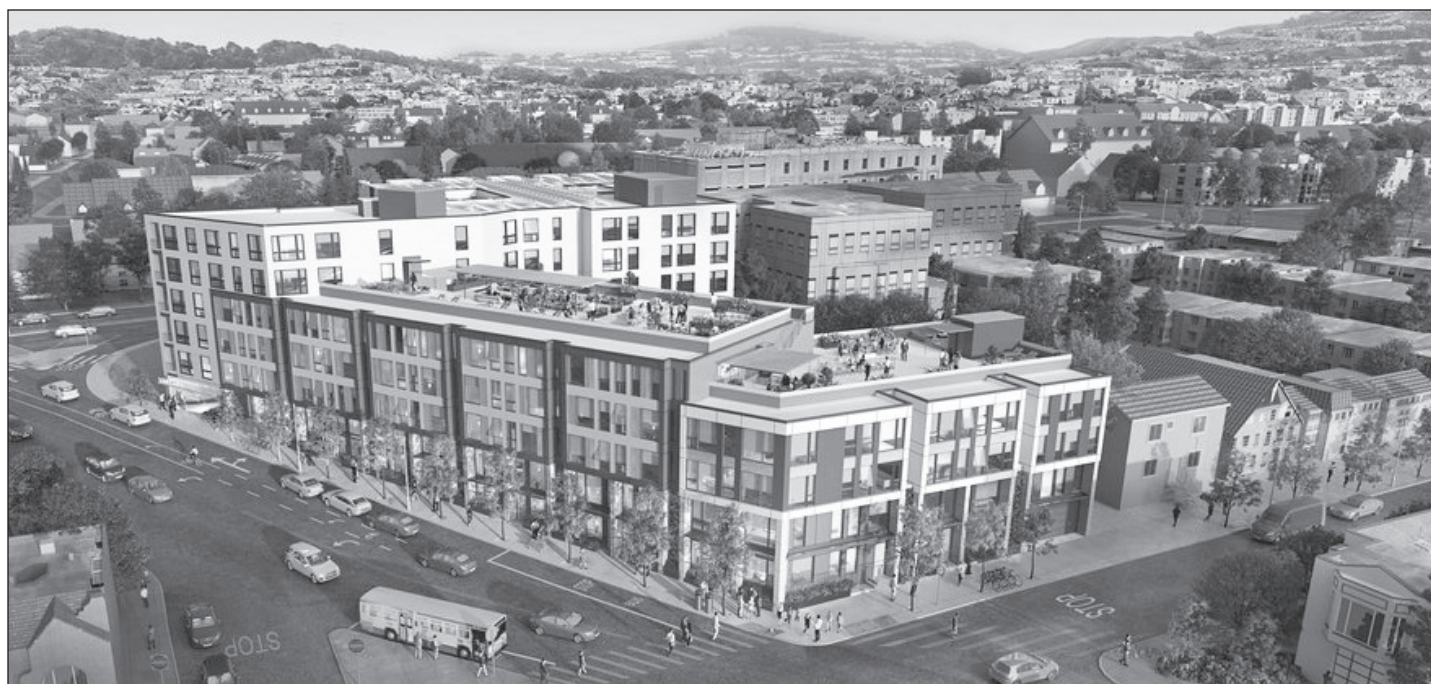
Groundbreaking for 99 Ocean Avenue expected this fall. The project will supply 193 housing units including 48 below-market-rate as well as about 500 union construction jobs.
