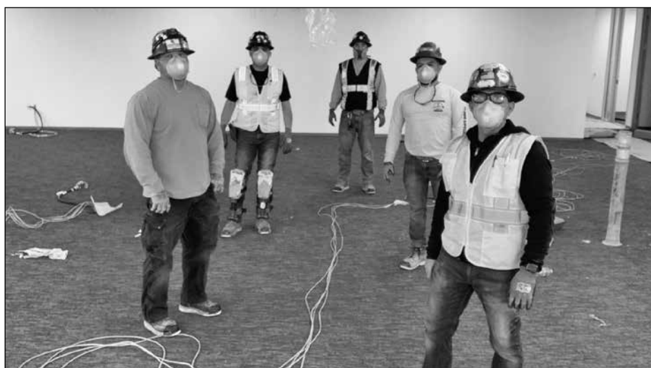
Andersons employees working while practicing safe social distancing.
