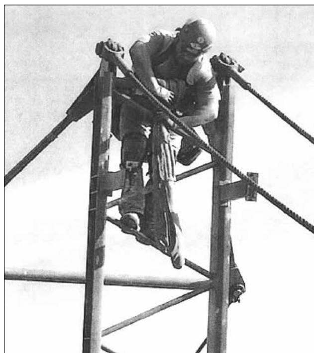
Martin R. Espinoza Jr. rigging in the crane with MCM – Tulare, CA 2016
