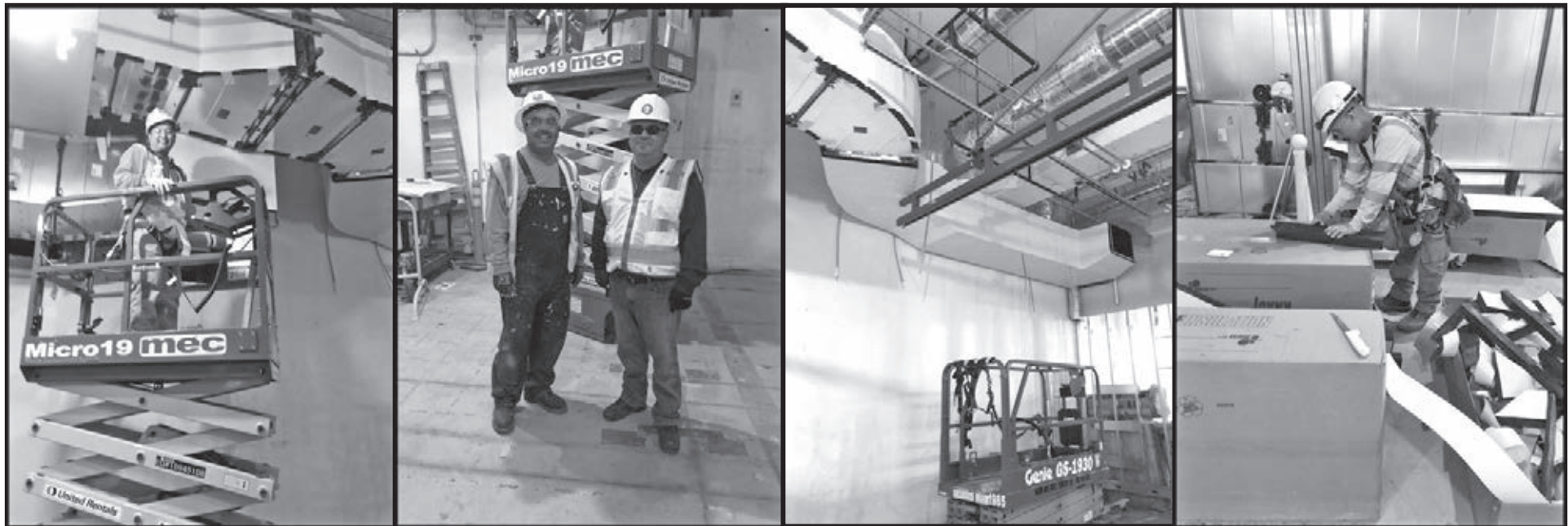
Local 16 members Carlos Diaz, Ariel Velasquez and Fernando Bautista working for Bayside Insulation Inc. insulating the ductwork and piping at Stanford.
