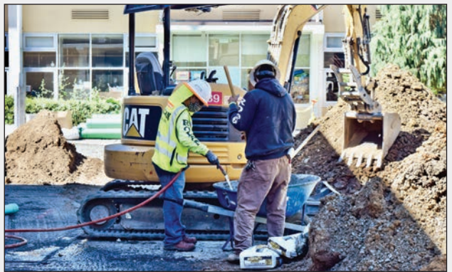
Rodan is the general contractor for the project at Clarendon Alternative Elementary School, which includes workers from several unions.
