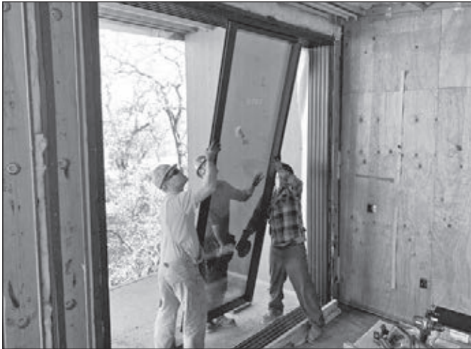
From left to right: Denver Miller, Casey Shepley, and Allen Brester in the picture installing a sliding unit at Montage in Healsberg.
