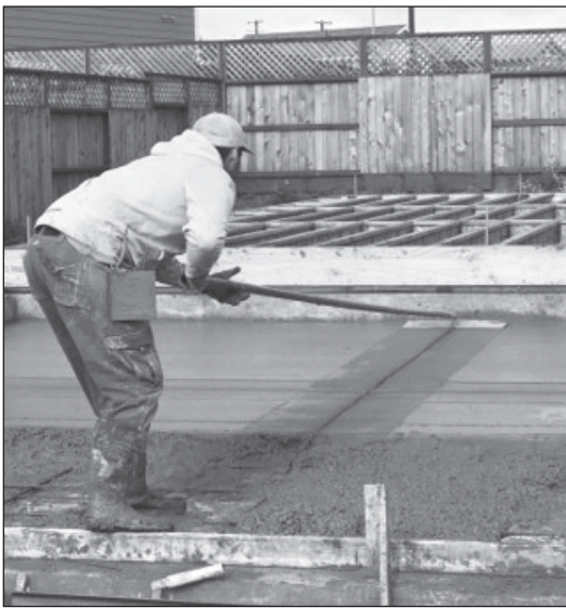
Local 300 Cement Mason apprentice Alex Rodriguez working in Santa Rosa.
