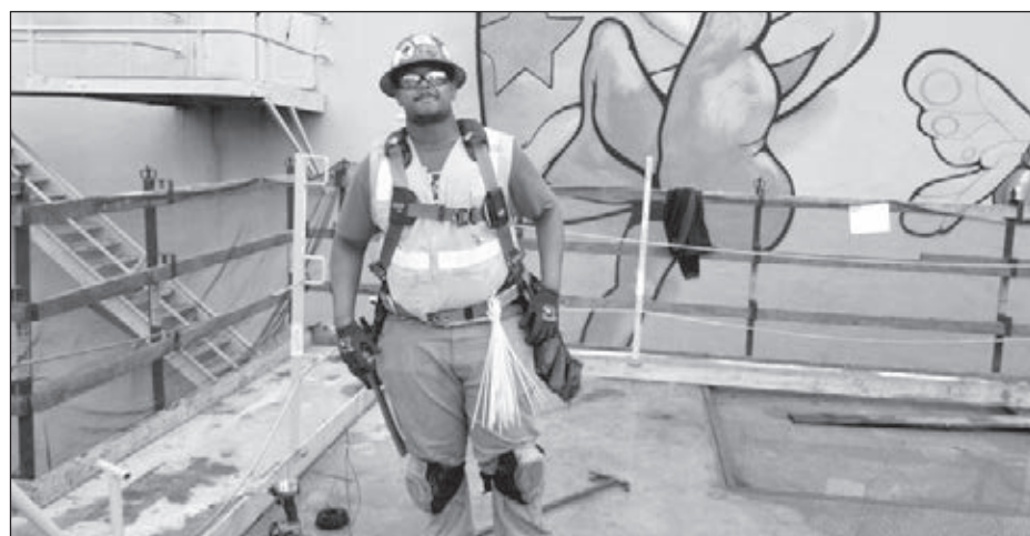
Mickey Manuel on the 950 Market Street job site.
