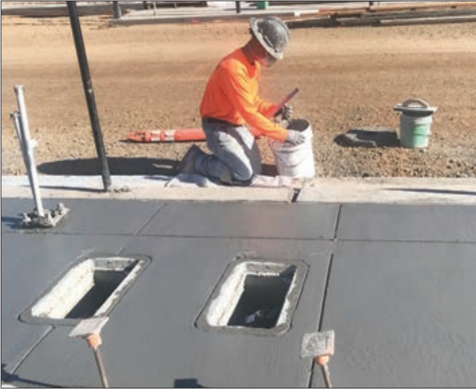
Local 300 Cement Mason apprentice Antonio Reinstadler patching curb at Sonoma Valley High School.
