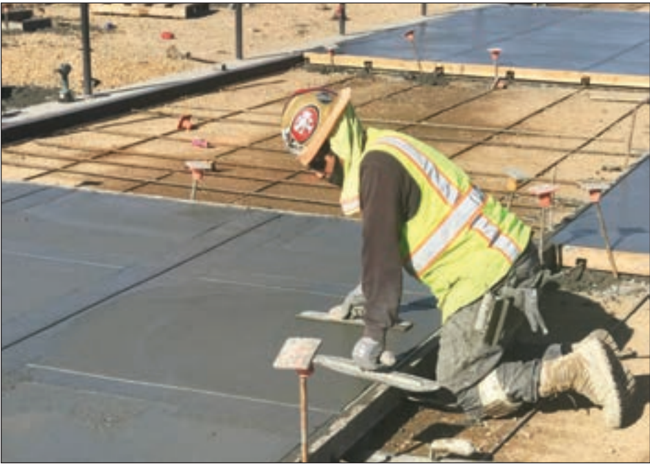
Local 300 Cement Mason Rafael Hernandez troweling flatwork at Sonoma Valley High School.
