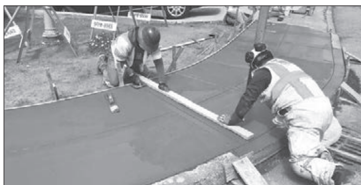
SF City and County Cement Masons pouring sidewalk in the Silver Terrace neighborhood.
