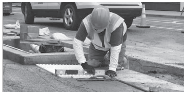
SF City and County Cement Masons improving path of travel on Bryant St.
