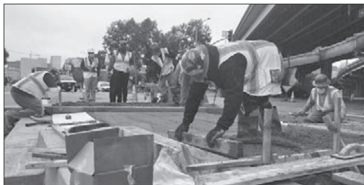
SF City and County Cement Masons improving path of travel on Bryant St.
