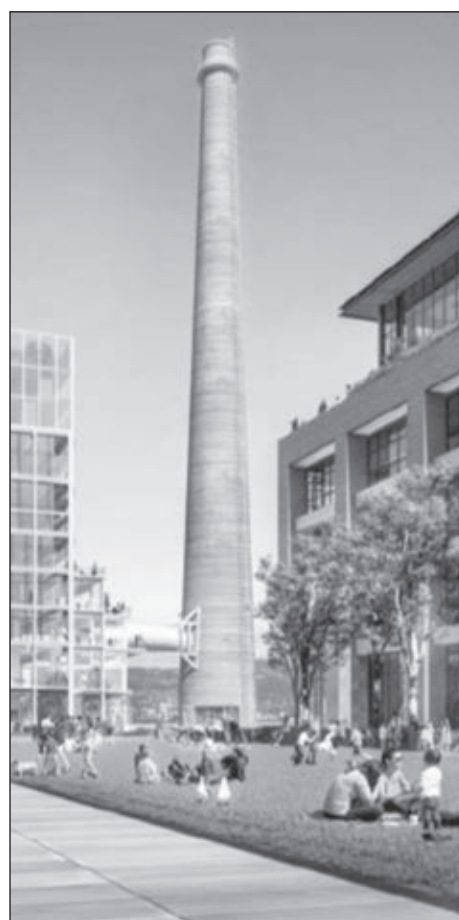
Potrero Power Plant
