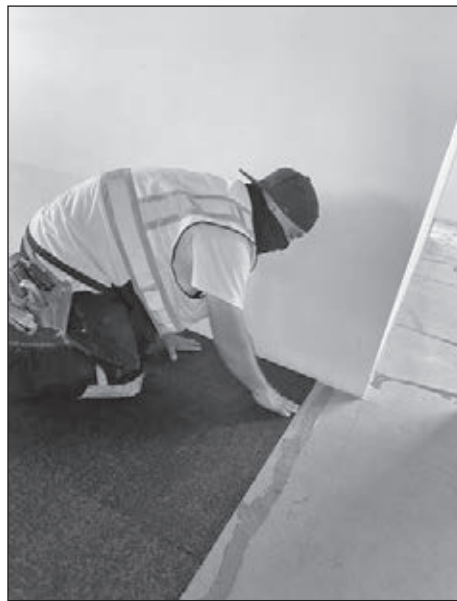
Daryl Katena (Above) and Mike Gabka ((Right) installing carpet tile for Pro Spectra.
