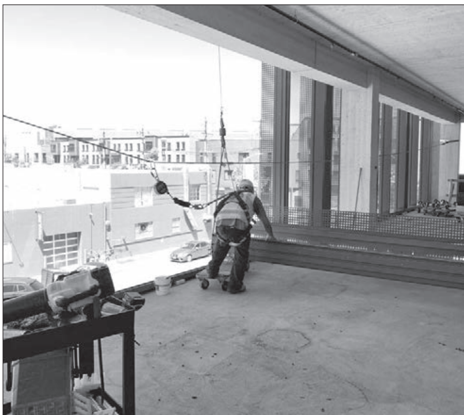
Top and above: Glaziers Local 718's Mike, Jerry and Horacio of AGA glazing 1 De Haro project.
