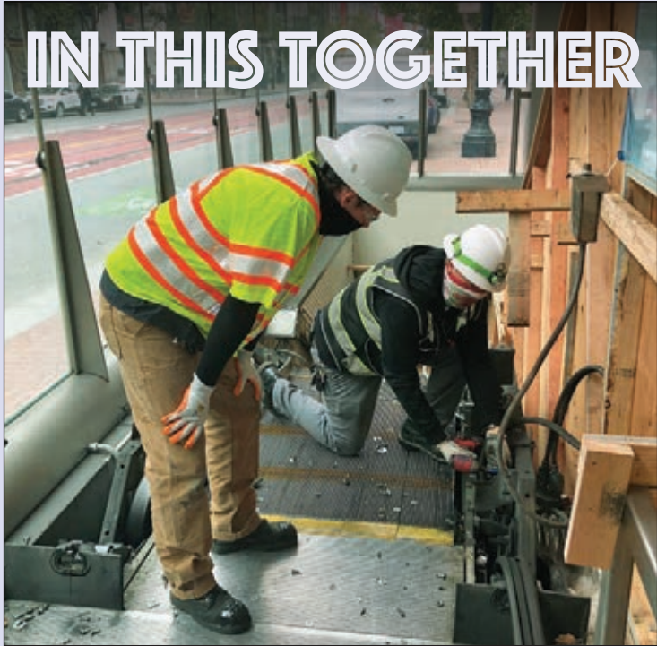
Elevator Constructors Local 8 mechanic Zach Jones with Apprentice Dylan Johnson on the jobsite.
