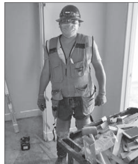
Dagoberto Flores on RT Western's Mission Bay job site.
