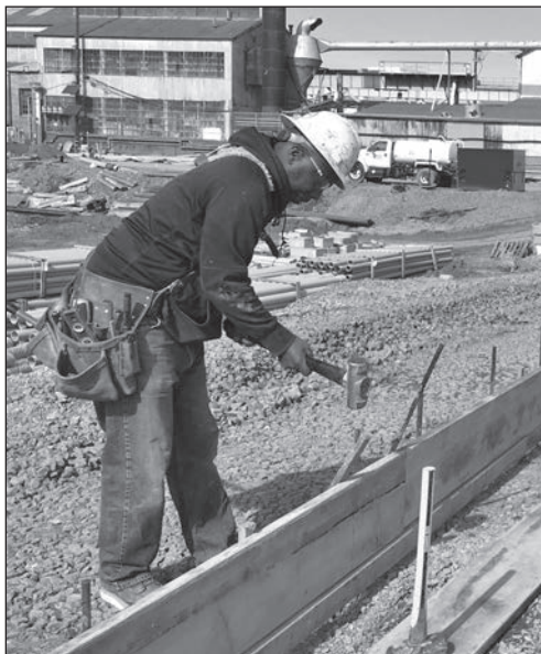
Local 300 Journeyman James Fox working with Bauman Landscaping, Pier 70 San Francisco.
