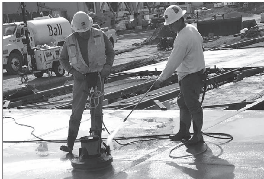
2 Local 300 Journeyman Cement Masons exposing concrete for Gordon Ball, Crane Cove project San Francisco.
